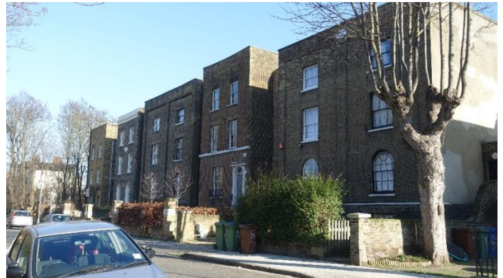
Figure 12 Late Georgian houses: Nos 47–59 Cobourg Road
