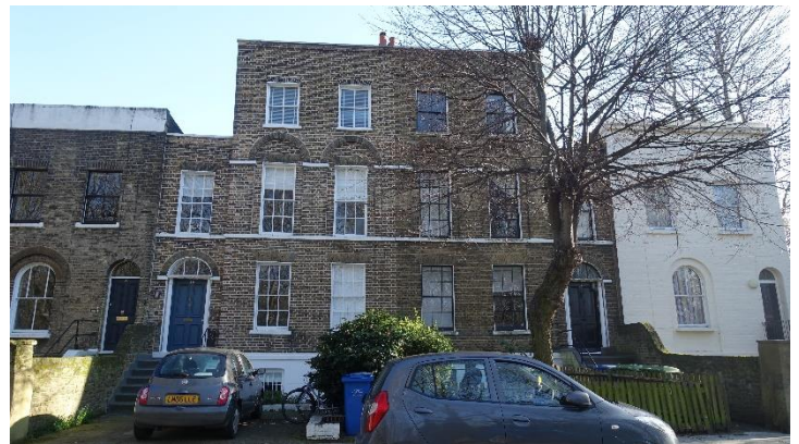
Figure 11 Nos 29–31 Cobourg Road. No.33 to the right.
