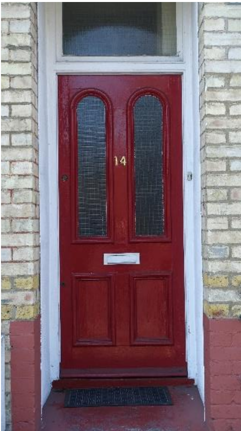
Figure 16 Original front door complete with bolection mouldings
