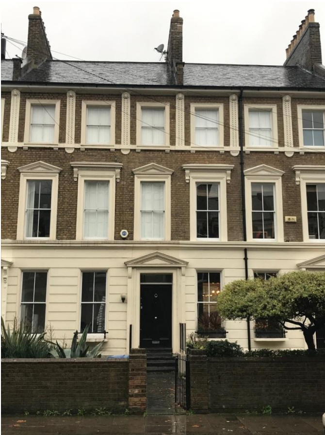
Figure 8 Detail of 16–24 Trafalgar Avenue
