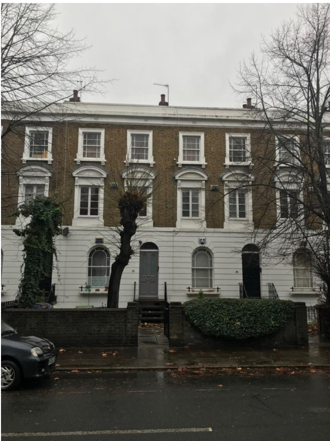
Figure 9 Detail of 42–48 Trafalgar Avenue
