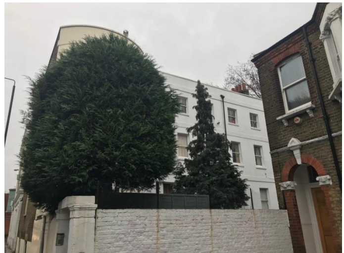
Figure 7 Nos 1 and 3 Trafalgar Avenue or Ship House, formally Ormond House
