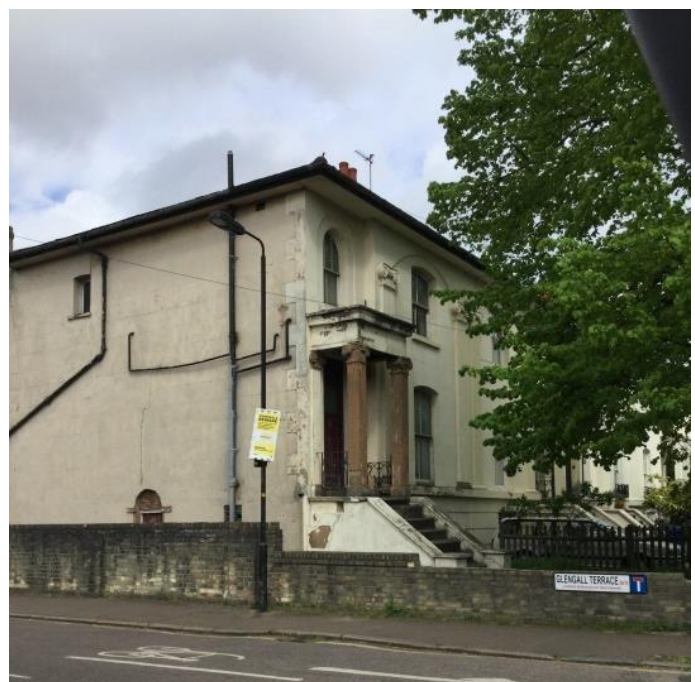
Figure 9 No. 38 Glengall Road
