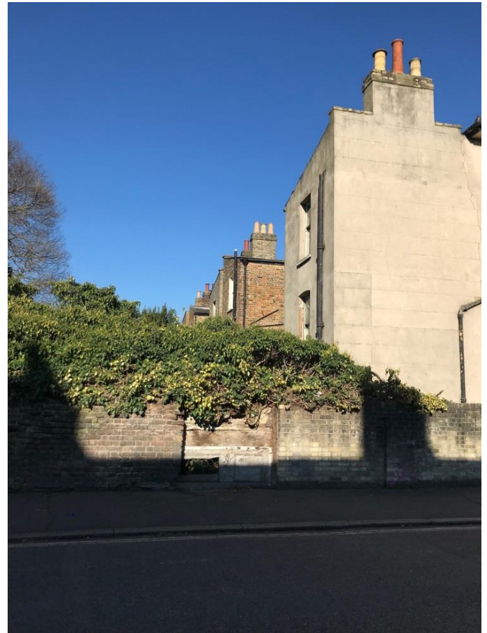
Figure 4 Rear elevations Nos 34, 36, 38 Glengall Terrace
