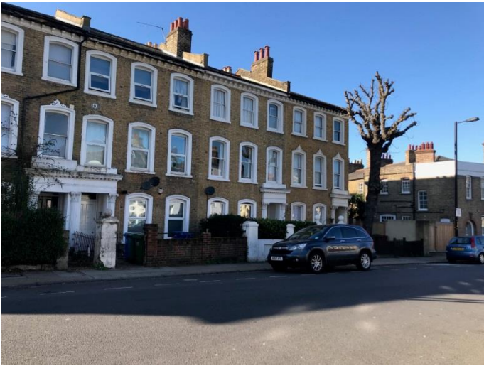
Figure 6 Nos 40–46 Glengall Road
