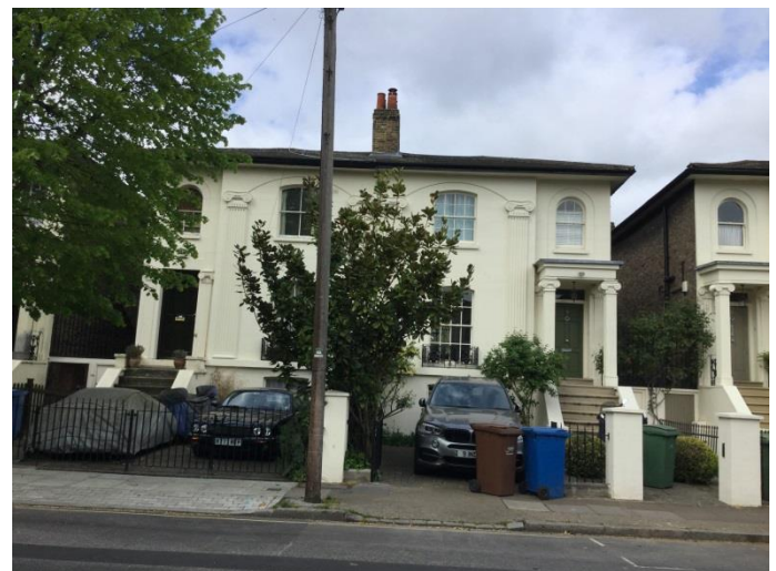
Figure 4 Nos 30, 32, 34 Glengall Road
