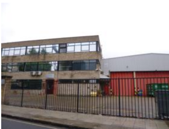
Figure 43 Galleywall Trading Estate
