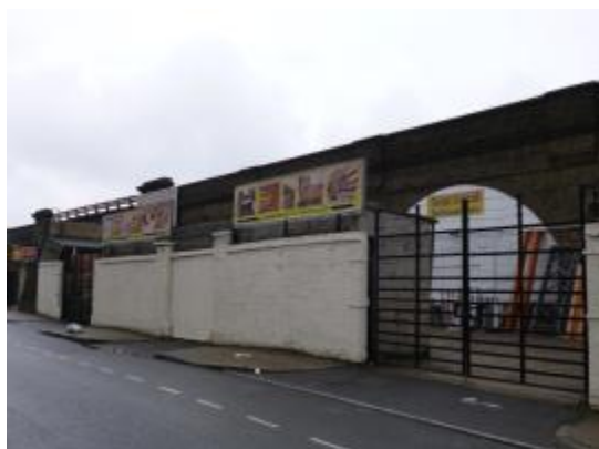
Figure 34 Raymouth Road Railway Arches
