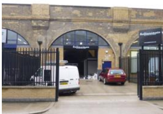
Figure 36 Raymouth Road Railway Arches
