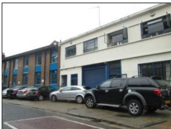
Figure 9: Capital Steel Site Services
