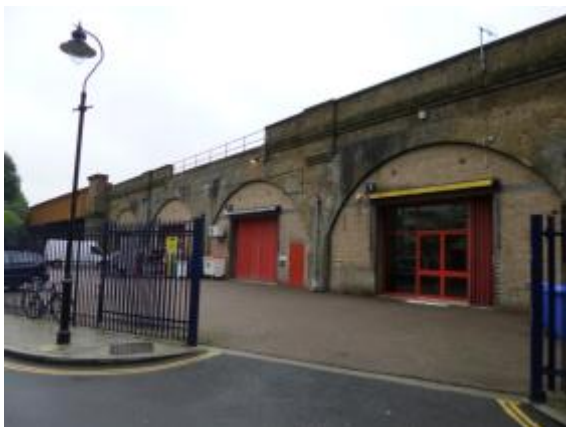
Figure 42 Clements Road Railway Arches
