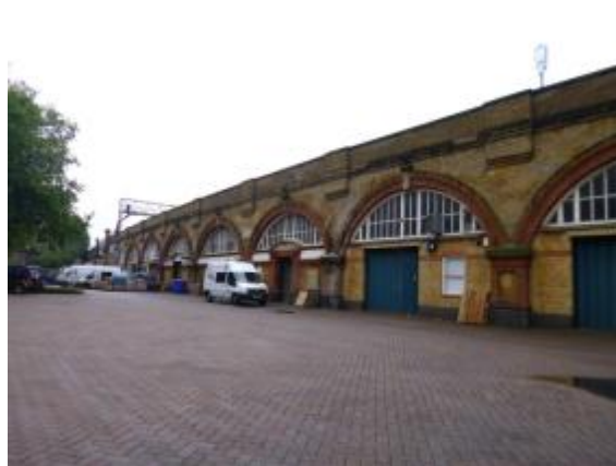
Figure 42 Clements Road Railway Arches
