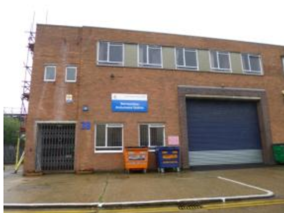
Figure 42 Bermondsey Ambulance Station
