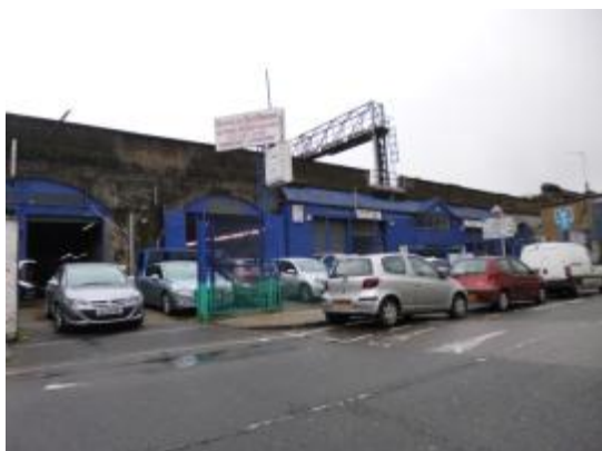
Figure 39 Raymouth Road Railway Arches
