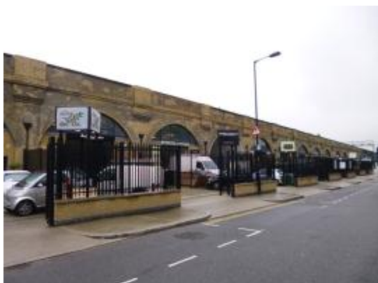
Figure 38 Raymouth Road Railway Arches
