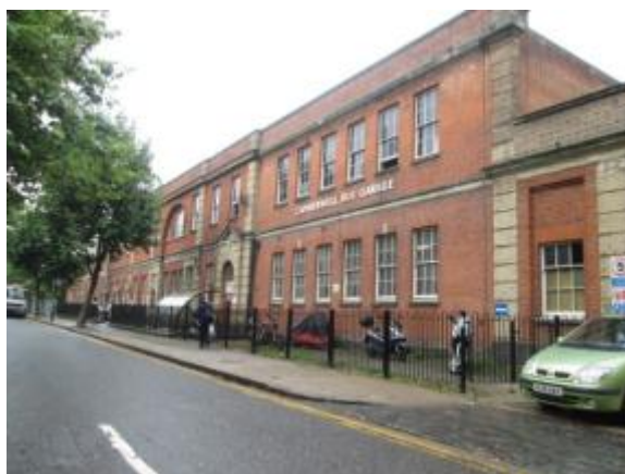
Figure 49 Camberwell Bus Garage
