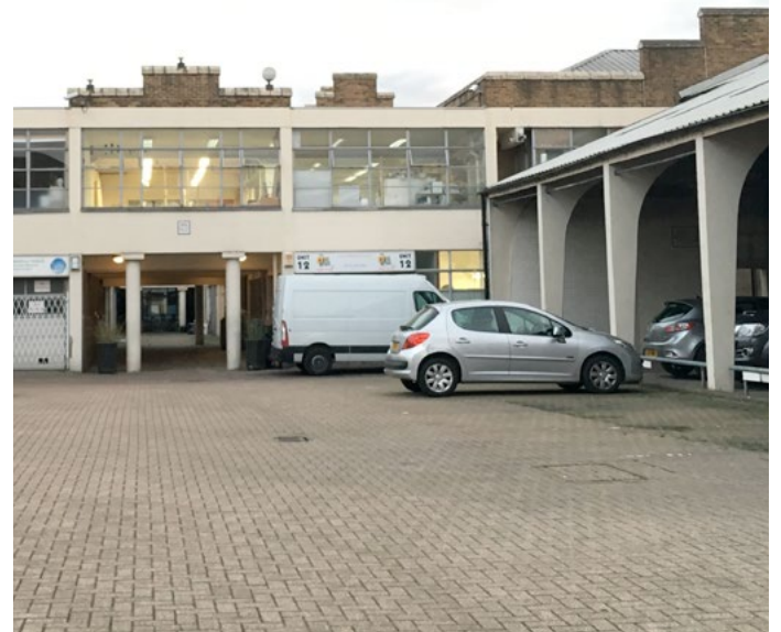
The OKR area is home to many small-scale food & drink, textile and fabrication businesses.
