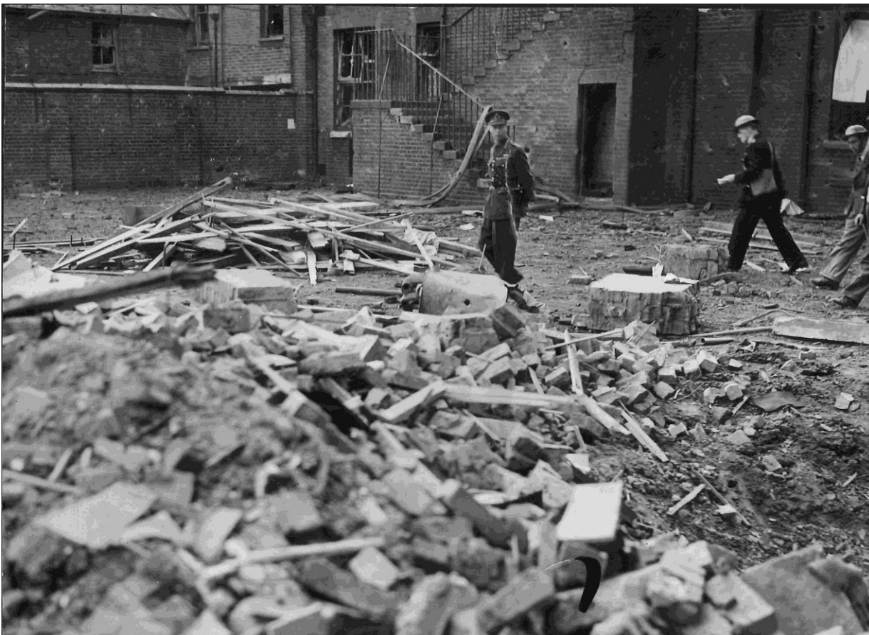
King George VI inspecting damage to Keeton's Road School, Bermondsey, shortly after 7 Sep 1940 From the image collection of Southwark Archives
