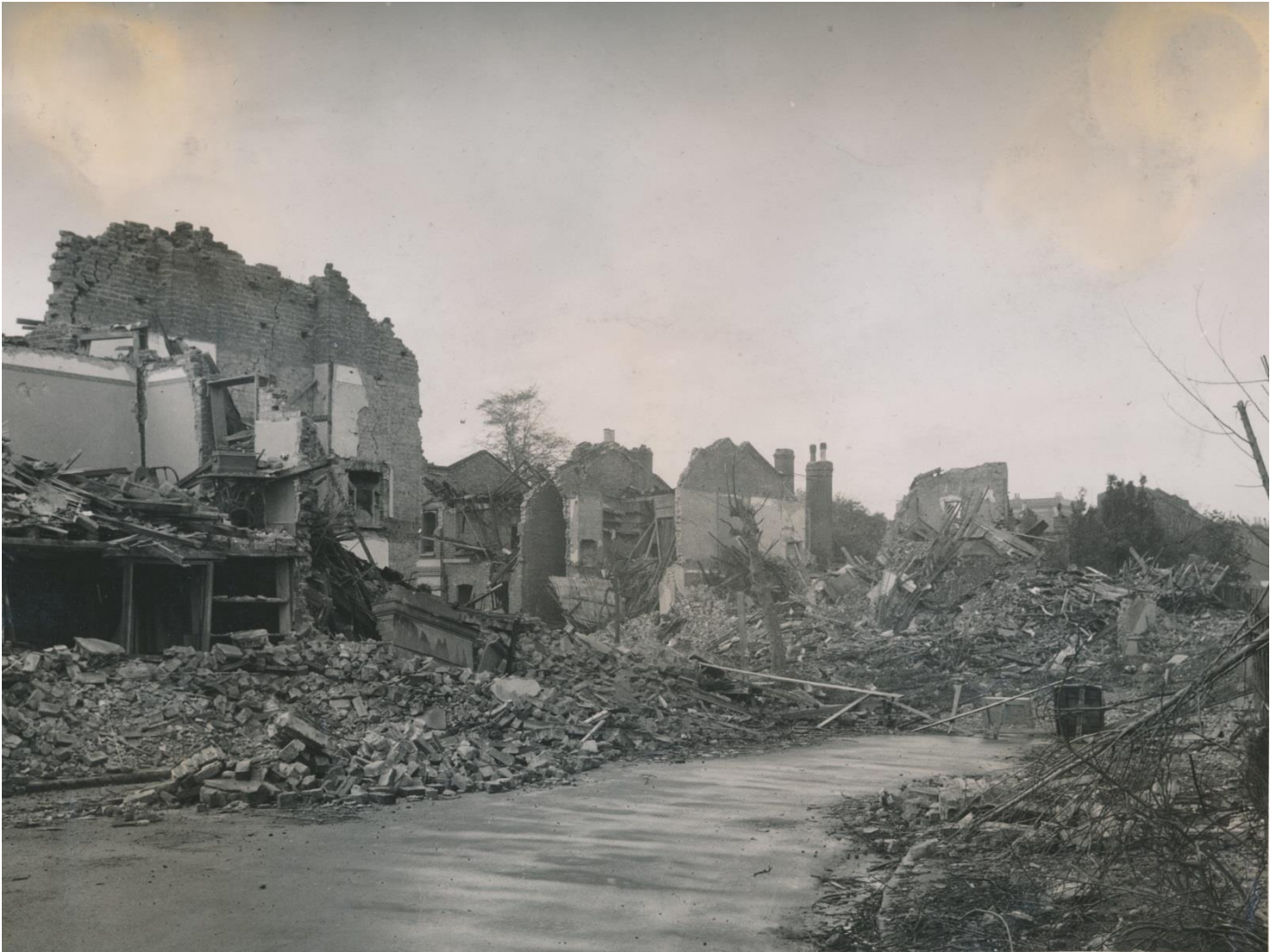
Damage from parachute mines, Camberwell, c 1943 (Photo by Barr): Southwark Archives image P 6922
