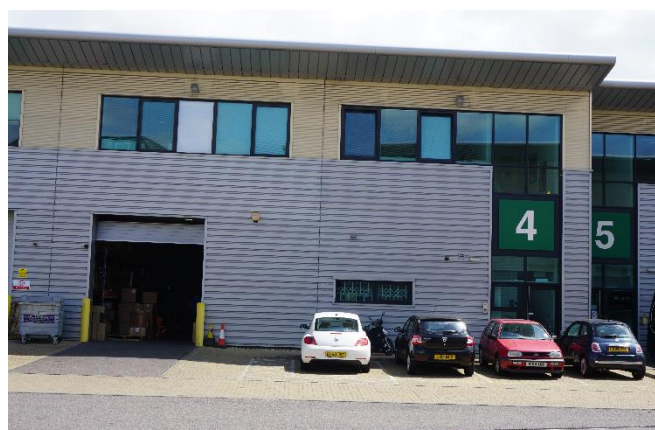
Figure 8.2 Glengall Business Centre Light Industrial Property
