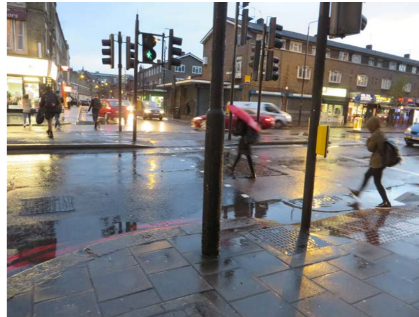
Evidence of poor maintenance of drainage affecting crossing facility
