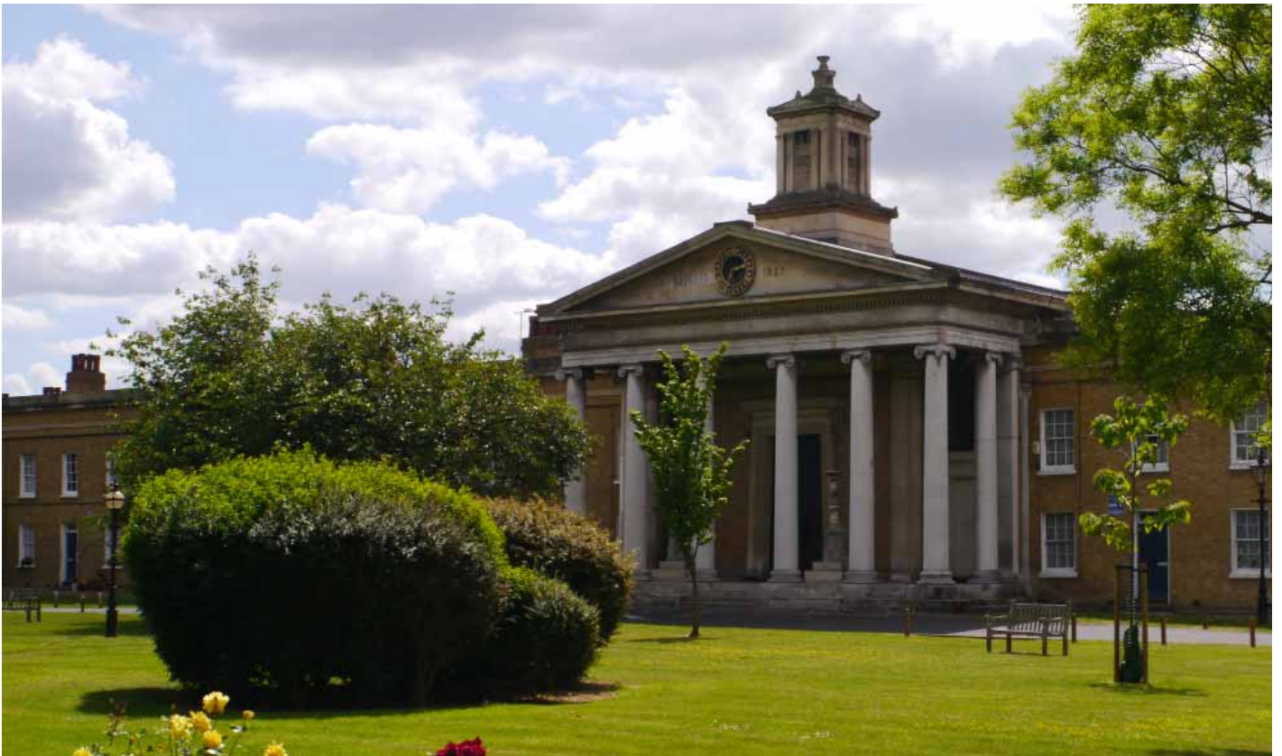
Caroline Gardens conservation area
