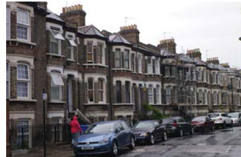
50 Madron Street Late Victorian terrace backing onto the main terrace of Old Kent Road. Three storeys with full height turreted bay windows. Brick with stone dressings, slate roofs and chimneys
