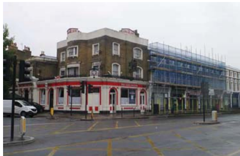
53 Old Kent Road / Trafalgar Avenue Consistent mid 19th Century range. Three storey block with stock brick, sash windows and Italianate detail. Ground floor contemporary shops with some detail retained such as console brackets. Butterfly roofs evident behind cornice line. Lord Nelson pub on corner.
