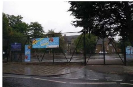
42 Boutcher Church of England Primary School Late Victorian school building in grey brick. The steep slate roofs and strong dormer windows lend it a gothic air. Set well back from the road with playground and chainlink fencing onto the pavement. Remains in use as a school and has been extended to the west.
