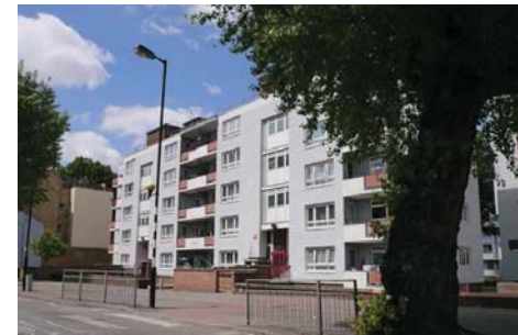
101 Rennie Estate Residential estate comprising towers, slabs and lower ranges at irregular angles. All in buff brick with white panels and flat roofs. Communal gardens and hard surfacing between the blocks.
