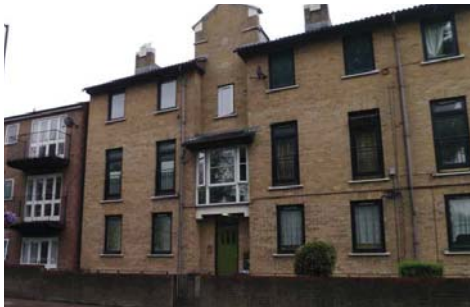
41 Grange Road south side. Three-storey flats, brick, deep plan, rear entrance from courtyard
