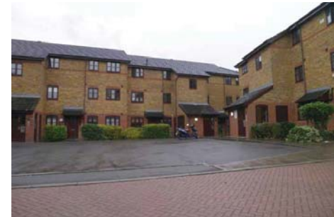
51 Buttermere Close Residential apartment blocks. Three storeys, yellow brick and dark tiles. Cul-de-sac layout with a central parking court and the buildings largely turning their back to the road. Late 1980s/early 1990s
