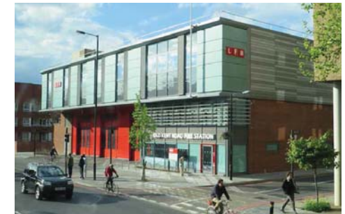
56 Old Kent Road Fire Station New Fire station built in 2015. Blue3 construction with BDP architects. Two storey unit with flat roof. Cantilevered upper floor with blue-green and grey panels contrasting with red for the engine bays below. Building set back a little further than adjacent properties.
