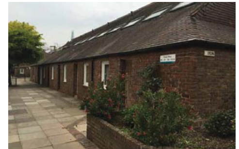
44 Curtis Street area Late 1970s Low rise modern terrace housing on a grid. Two storeys with attics, parking courts and mews-type development. Red brick and render, tile roofs
