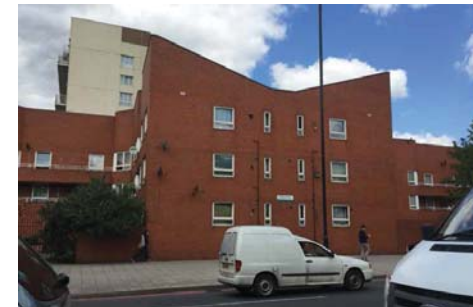
55 Wessex House Three storey residential blocks in U shapes on to the Old Kent Road. Dating from c 1970s with rear deck access. Red brick.
