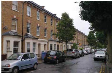
49 Marcia Road Late Victorian terrace (after 1871) on the site of the former goods yard stables. Three stories, stock brick, bay windows with stucco ornament and corbelled eaves. High level of consistency along the group.
