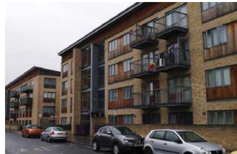
68 Cooper's Road Estate
