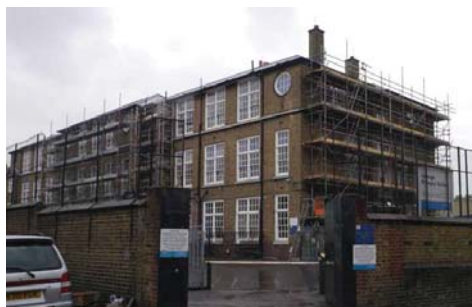
21 Webb Street School Typical Victorian school building set within playgrounds. Stock brick, slate roofs, three storeys c1900. This building remains in use as a school.
