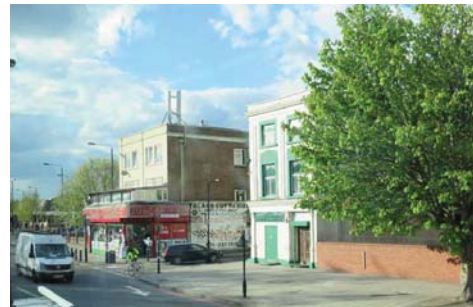
54 Old Kent Road / Rowcross Street Two Victorian remnants. Late Victorian three storey commercial block to the east with painted facades with some stonework detail. The frontage suggests that this was formerly a public house. The western block dates from the mid 19th Century with later shopfronts and extensions. It has painted brickwork and some period detail such as pilasters.
