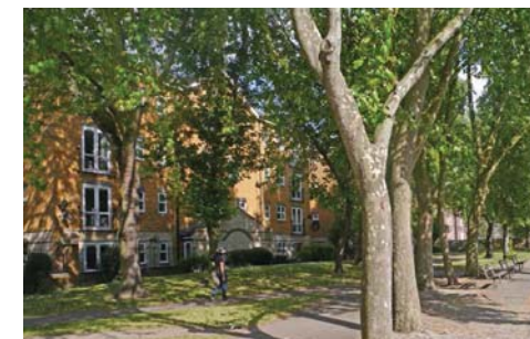
24 Old Kent Road Four-storey late twentieth century flat blocks set back from Old Kent Road behind trees. Pavilion form, yellow brick, dark hipped roofs. Predominantly accessed from the rear.
