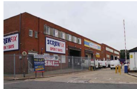
100 Bermondsey Trading Estate and South Bermondsey Railway Station Three-storey office units fronting wide span medium scale industrial units, mostly backing onto the railway viaduct. Developed c 1950s. Four turn of the century houses amid the rail lines are a remnant of a former terrace on Rotherhithe New Road.
