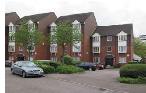
93 Sheppard Drive and environs Three and four storey residential blocks, irregularly clustered with parking courts and shared gardens. Grey and brown brick with hipped roofs. Dates from c 1970s and 80s.
