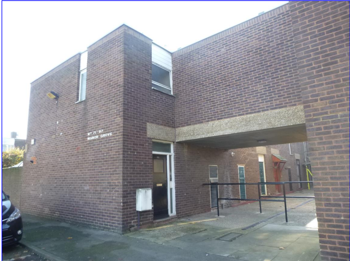
Photograph 1: General view of one of the Manor Grove terraced houses, at an end.
