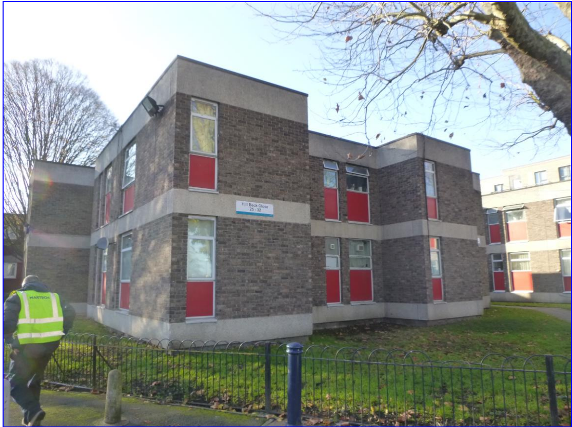
Photograph 6: General view of part of Hill Beck House.
