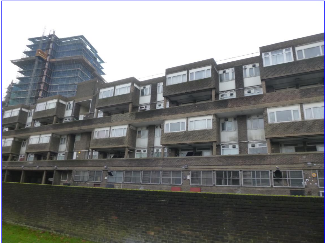
Photograph 4: General view of part of Bowness House (rear).
