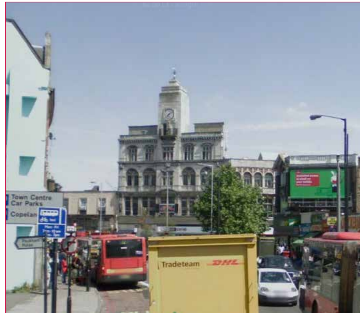
Former Jones and Higgins Dept Store façade with clock tower
