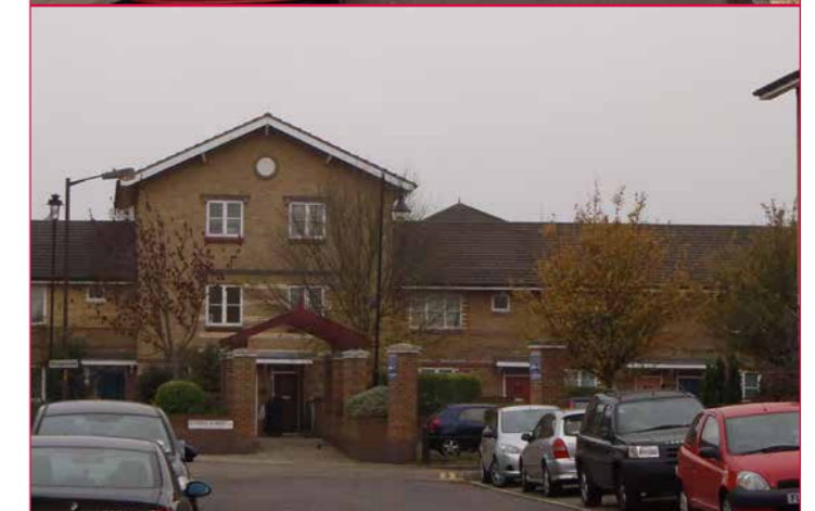
Examples of typical perimeter block development within the area: yellow brick, terrace houses with block of flats in corner locations, on-street and in curtilage parking
