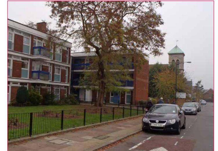
Glengall Road, Celestial Church of Christ creates a positive landmark in the area
