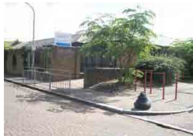
View outside the entrance to St John RC Primary School
