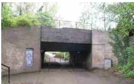
The Nelson Walk underpass looking west
