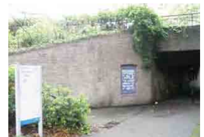
The Nelson Walk underpass looking east
