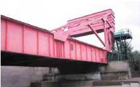
The Bascule bridge feature at the west end of Greenland Dock
