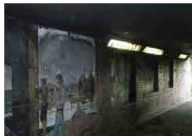
The interior of Nelson Walk underpass
