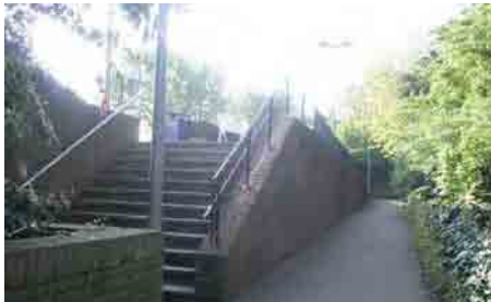
The existing stepped and ramped access joining the car park at Surrey Quays
