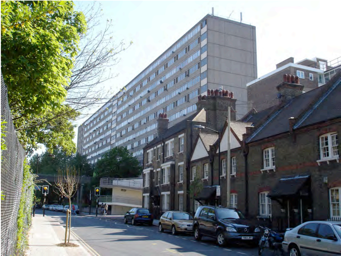
View 5. Portland Street north of junction with Hopwood Road looking south.
