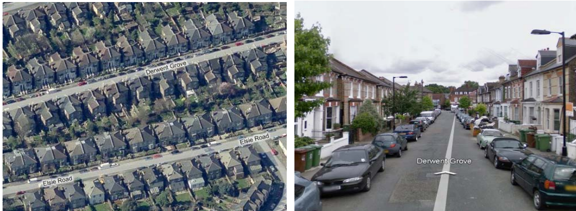
Block 8. Derwent Grove: Predominantly semi-detached housing. Approximately 81 dwellings per hectare.
