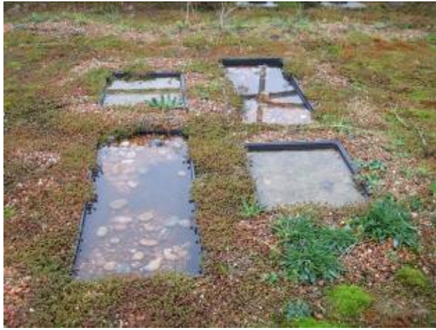
Green roof with water feature
