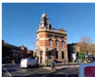
PROMINENT CORNER BUILDINGS
