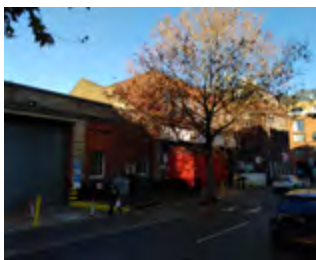
BRICK BUS GARAGES
