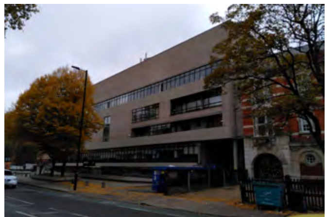
Above: University of Arts Extension, Murray Ward & Partners Completed 1960
