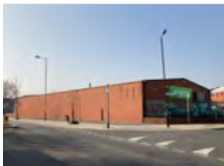
BRICK INDUSTRIAL BUILDINGS
