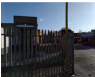
STEEL PALISADE FENCING
