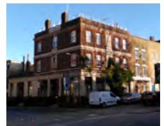
PROMINENT CORNER BUILDINGS
