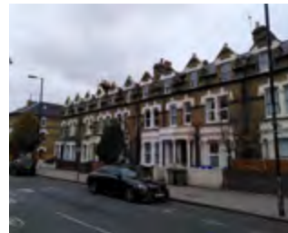
REGULAR BRICK FRONTAGES
