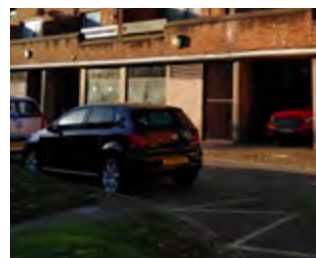
GROUND FLOOR GARAGE SPACE
