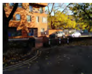
EXTENSIVE ACCESS ROAD NETWORK
