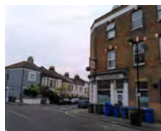
PROMINENT CORNER BUILDINGS
