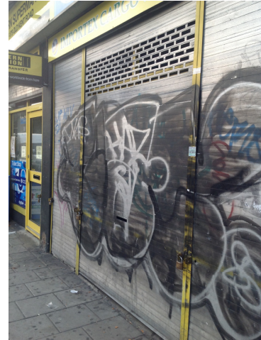
Figure 14: External roller shutters
