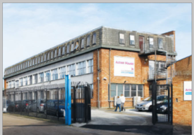
53 Sandgate Street (Site 1)
