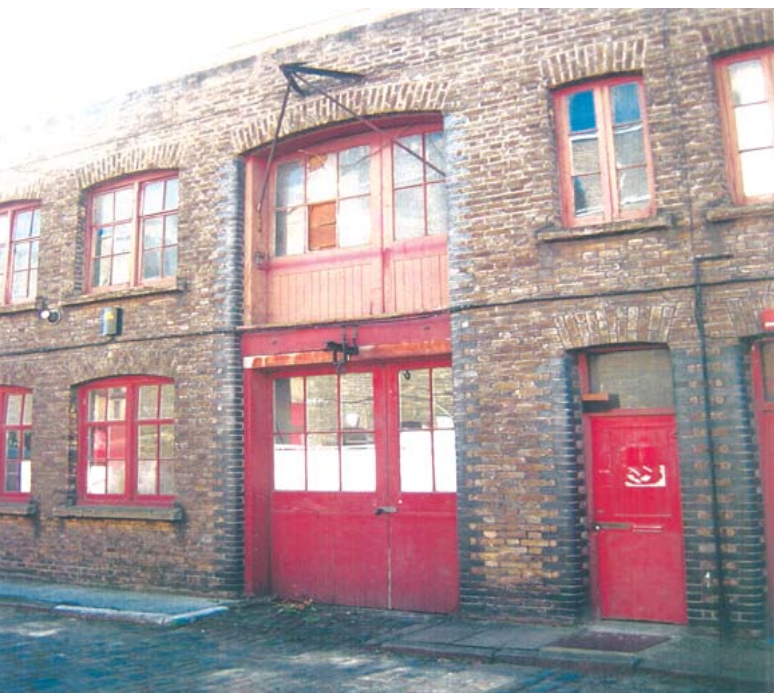
Figure 11: Detail of workshop elevation in Iliffe Yard.
