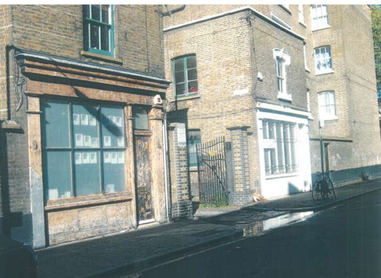
Figure 12: Shop fronts at the entrance to Peacock Yard.
