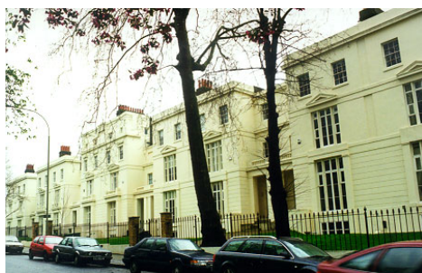
Figure 5 200-218 Camberwell Grove – recently renovated
