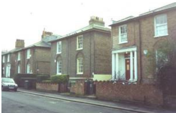
Figure 2 Semi-detached and terraced houses on Holly Grove continue to enjoy aspects onto the amenity space known as The Shrubbery.
