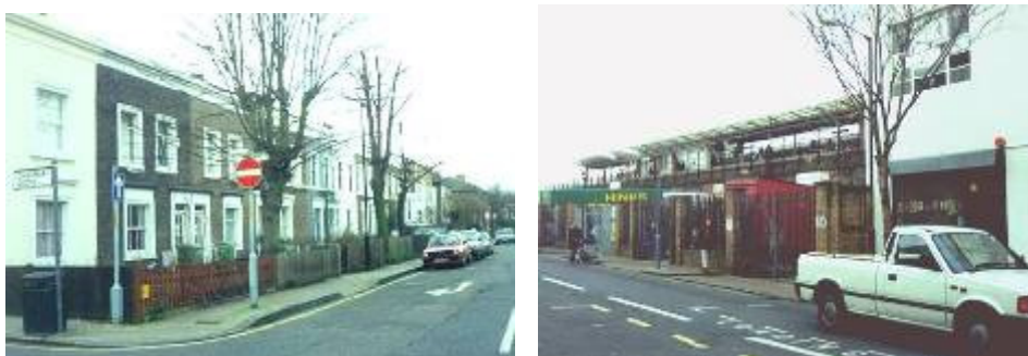
Figure 17 The good quality 19 th century housing on the south side of Blenheim Grove (left) is compromised by the light industrial uses on the north side of the road (right) and some insensitive infill development.
