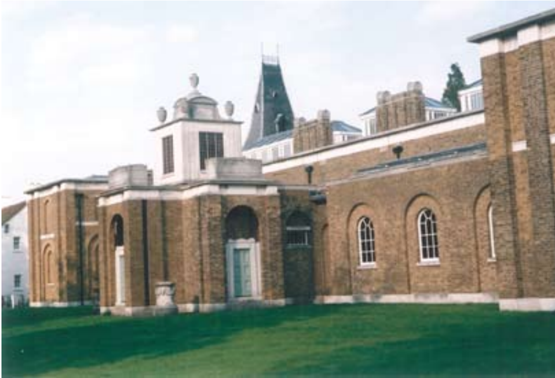
Figure 10: The Dulwich Picture Gallery from Gallery Road.
