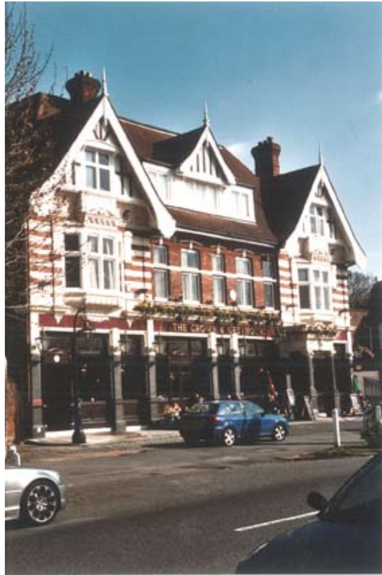
Figure 15: The Crown and Greyhound public house, Dulwich Village.
