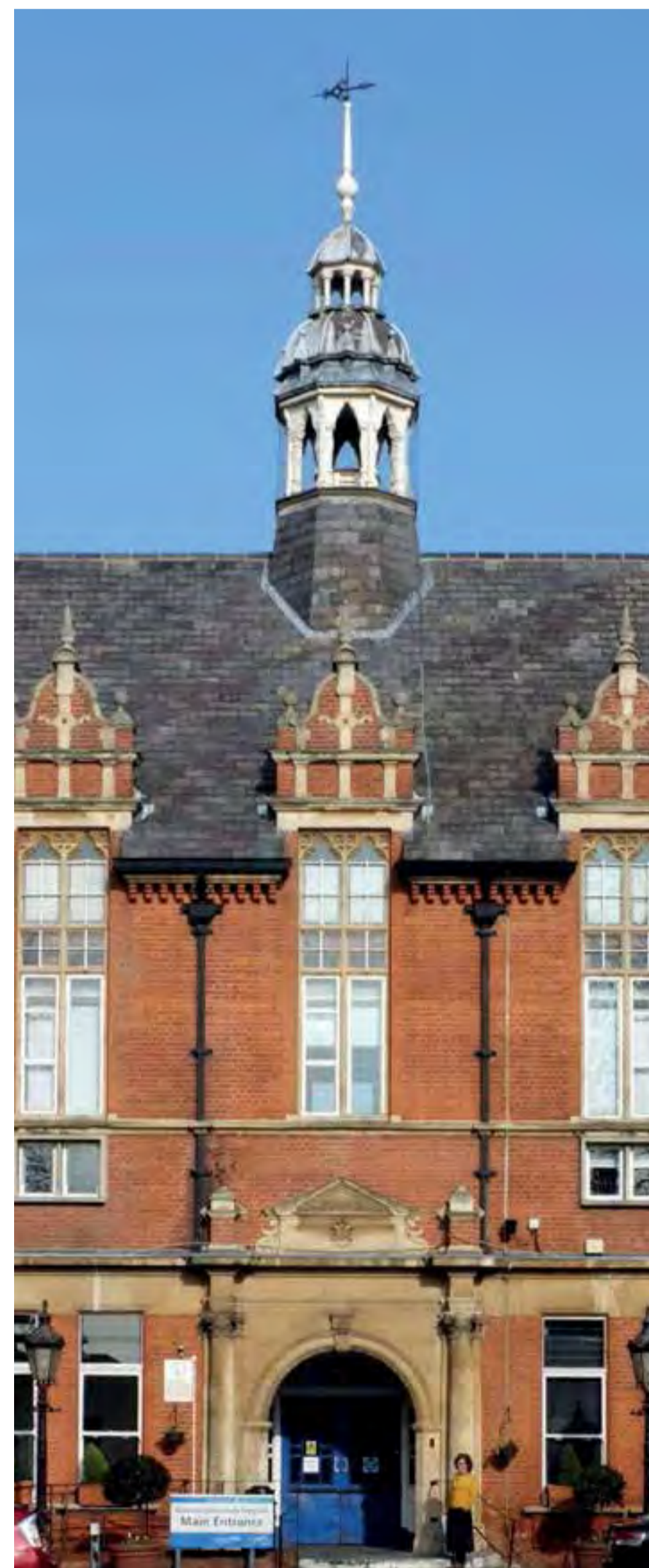
Existing Site Materials
