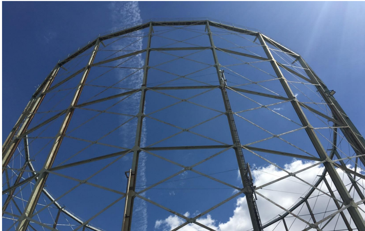
Detail of the gasometer
