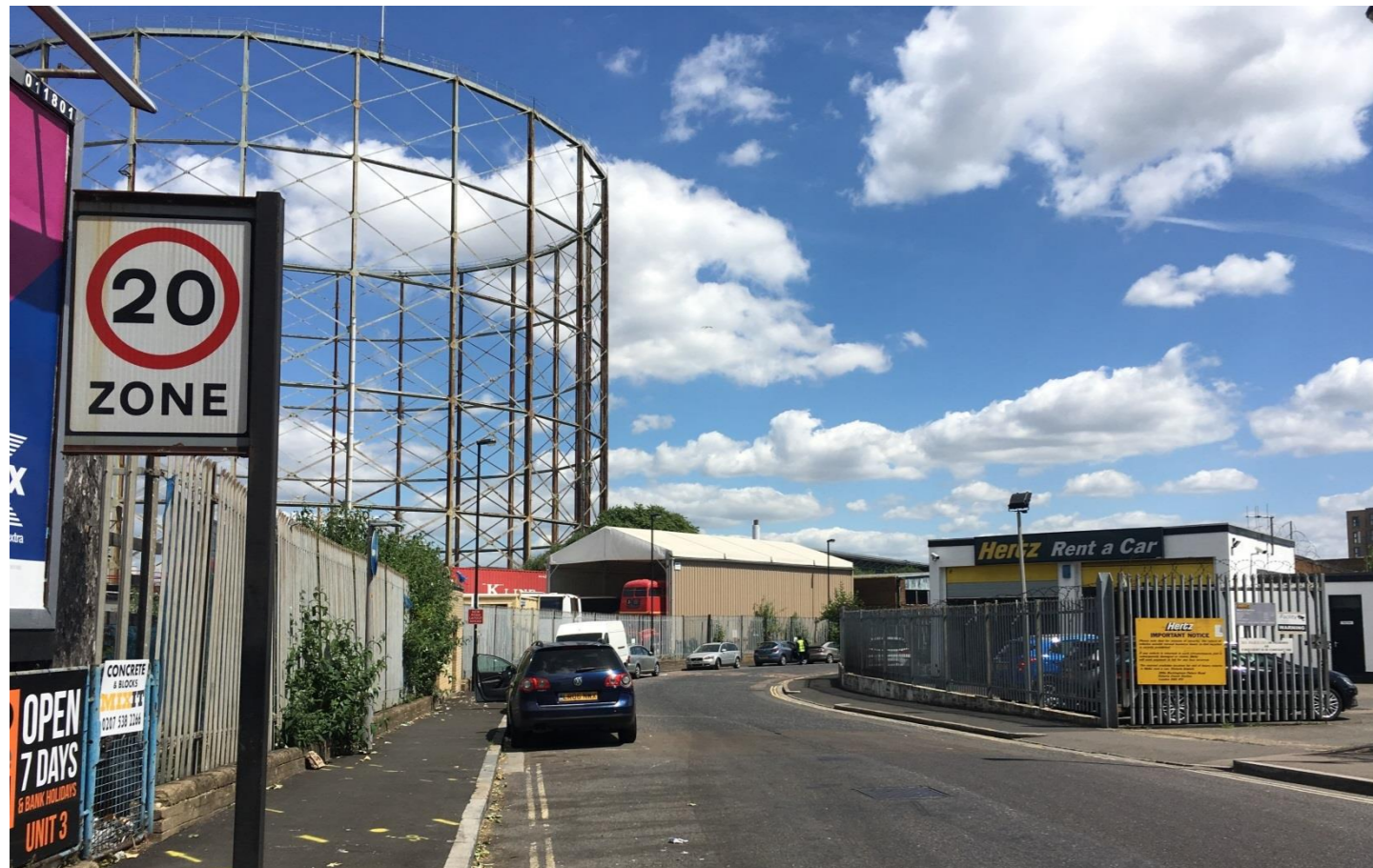
Entrance to Devon Street from Old Kent Road
