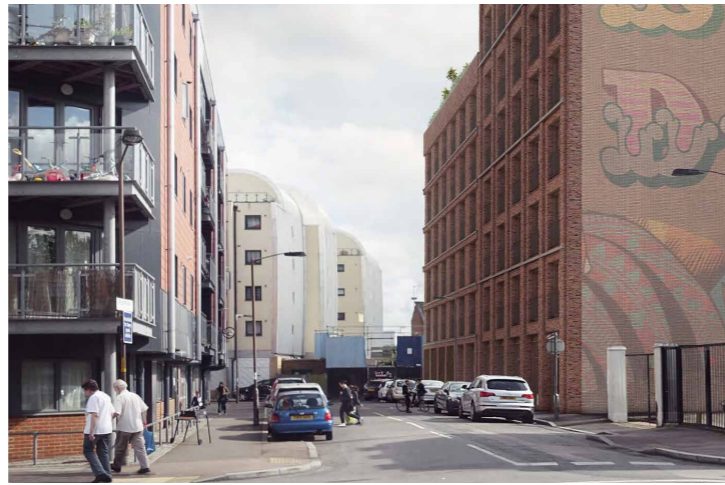
B. 1 Varcoe Road: Planning permission granted for a mixed use development up to 8 storeys including 57 homes and workspace on the ground floor. (Planning ref: 16/AP/5235). Currently under construction.
