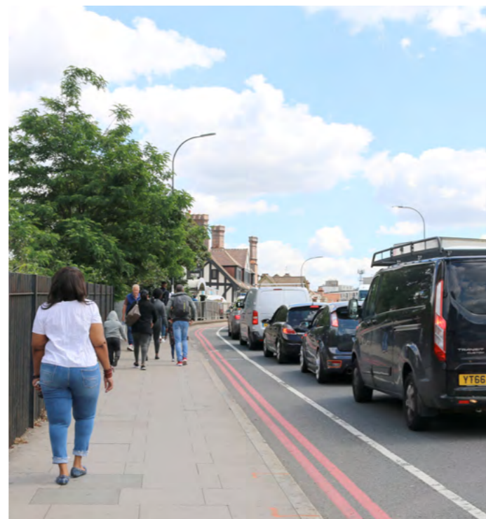
There is potential to increase pedestrian paths add more crossings along the rail bridge by extending the rail bridge to the south.
