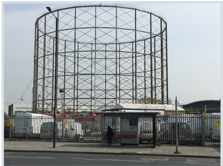
Old Kent Road gas tower
