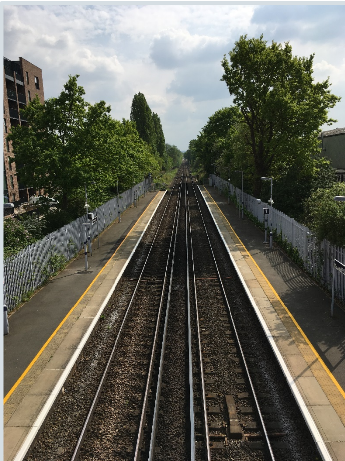
Lower Sydenham station
