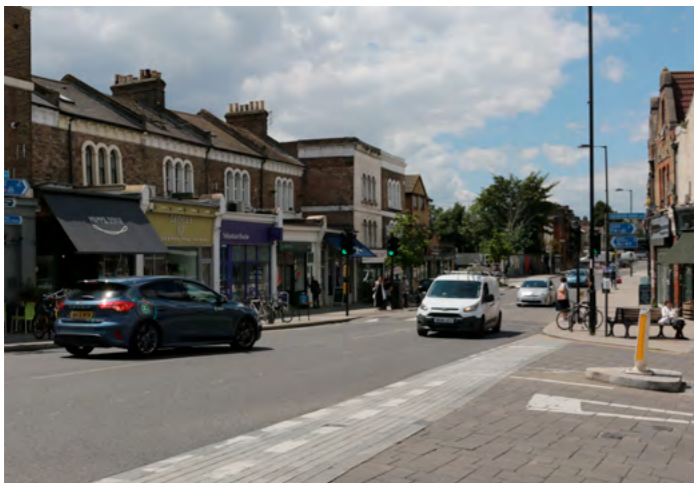
Existing raised tables to assist pedestrian movements across side roads could see reductions in corner radii to reduce traffic speeds and crossing times.
