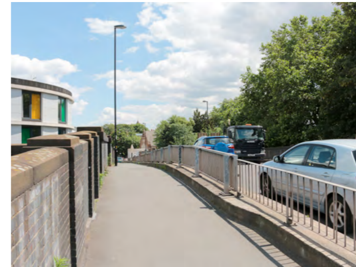
Railway and Ravensbourne River create east-west severance, navigated by the tall highway bridge. Potential to improve crossing access and cyclability.
