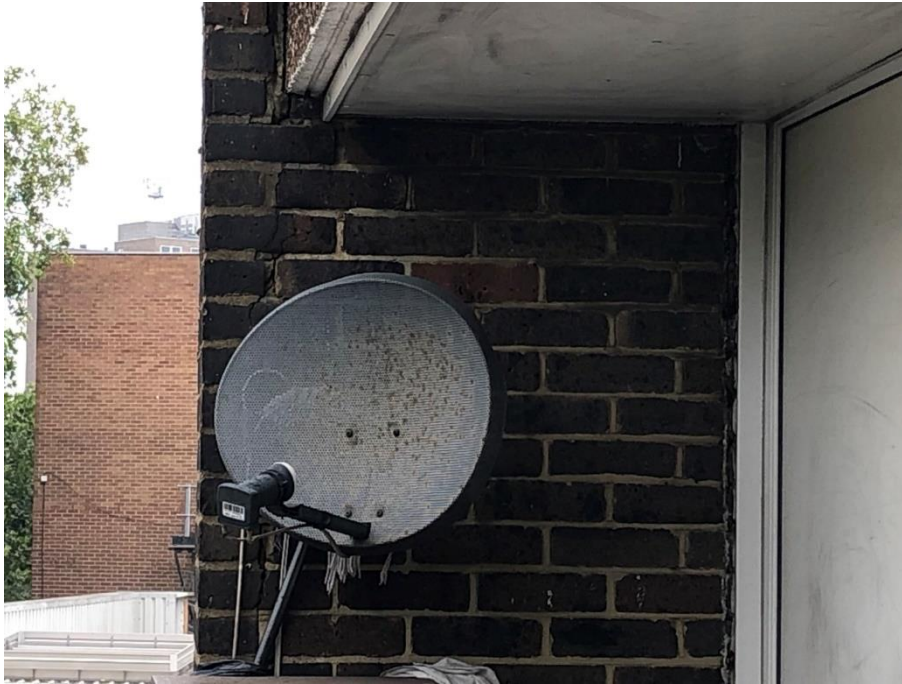
Photograph 9 – Bowness House – Vertical cracking to external brickwork at second floor level.
