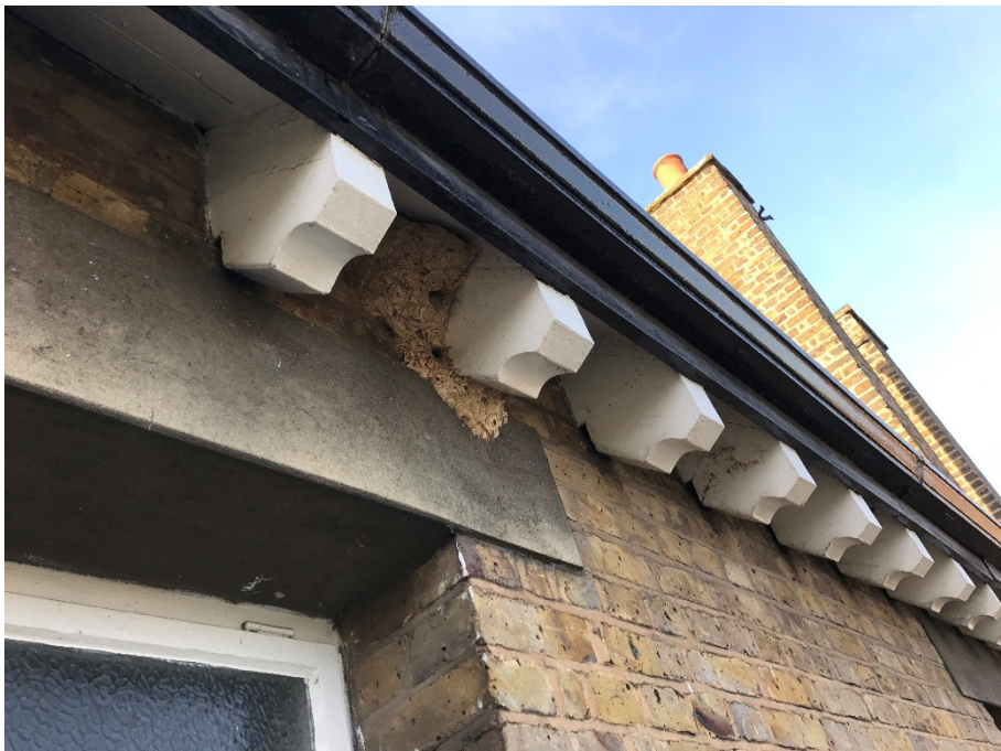
8. Eaves Detail to East Elevation
