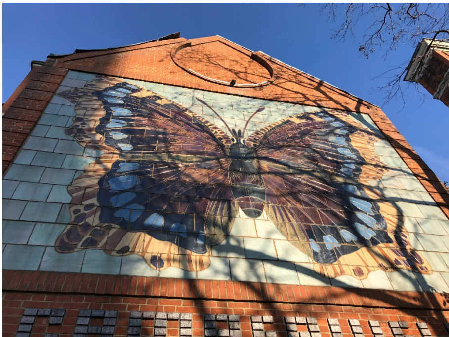
6. Tile Work to South Elevation
