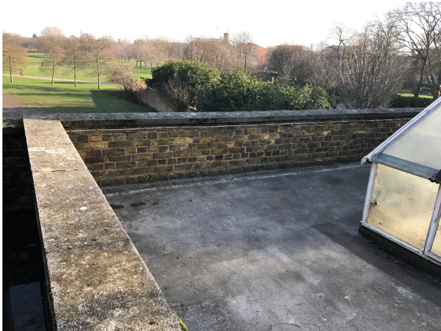
10. Parapet Wall to East Elevation
