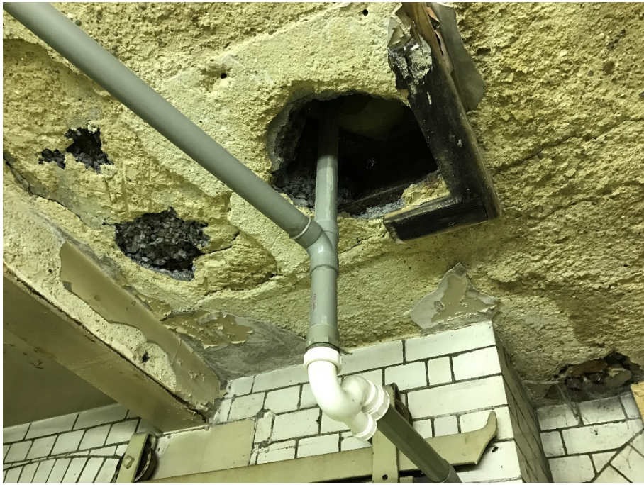
13. Basement Ceiling Slab
