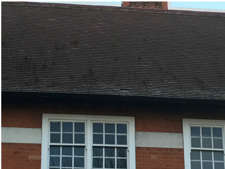
5. Tile Roof to West Elevation
