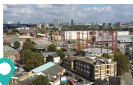
Gas works today
