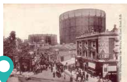
Old gas works
