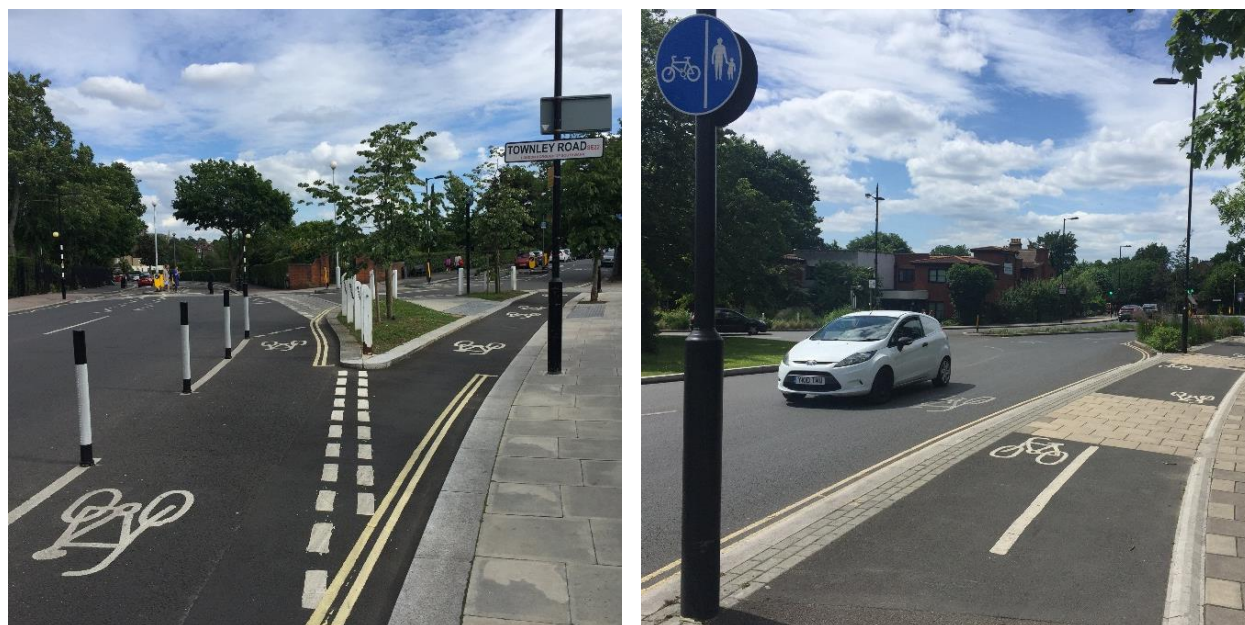
Figure 6.3: Cycle facilities along the future Quietway 7 route at Townley Road and Dulwich Wood Park
