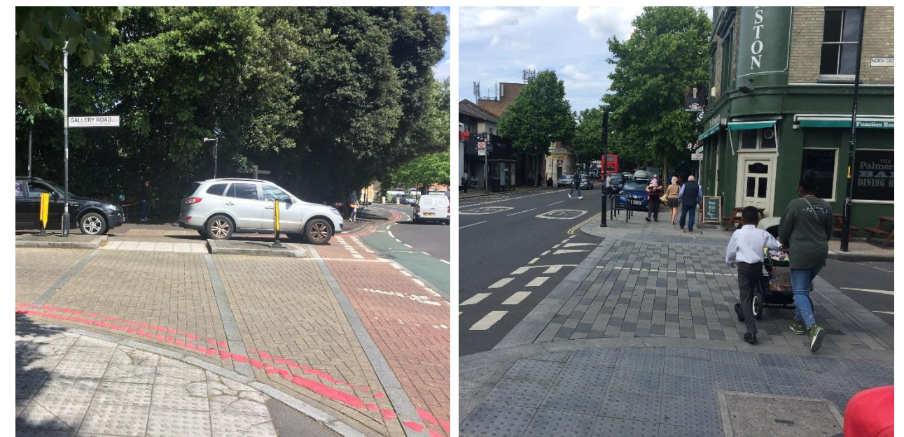
Figure 7.3: Raised Treatment at junction Dulwich Common/Gallery Road; raised side road entry treatments along Lordship Lane
