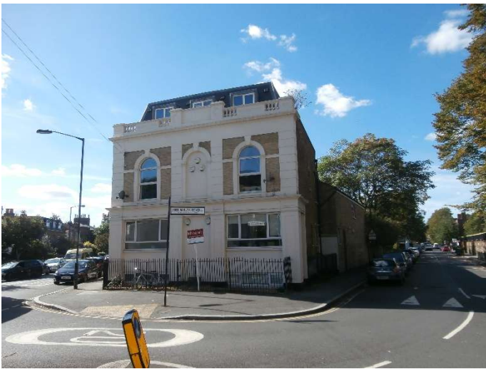
Figure 7 The former Sidmouth Arms public house.
