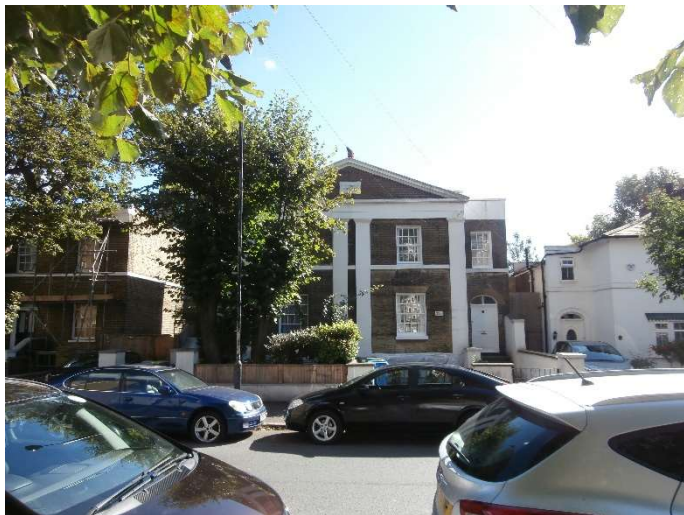
Figure 10 Doddington Cottages, Commercial Way
