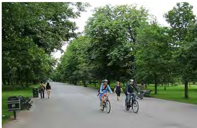
Fig. 1.71 Tarmacadam paving The Broadwalk, Regents Park
