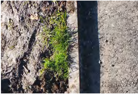
Fig. 1.9 Concrete pin kerb
