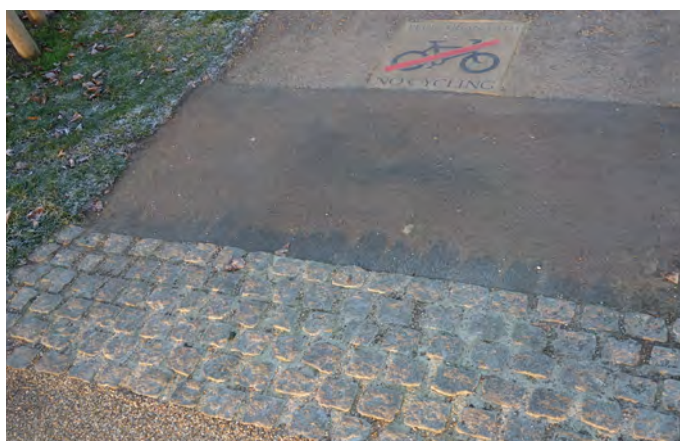
Fig. 1.72 Granite setts at junction, Hyde Park
