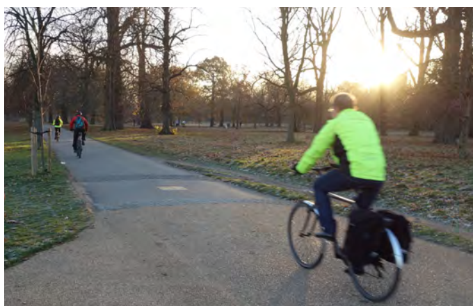
Fig. 1.73 - Spray and chip surfacing at junction, Kensington Gardens
