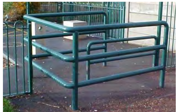
Fig. 1.37 - Typical motorcycle entrance/exit barrier
