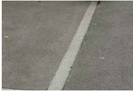
Fig. 1.10 Granite Kerb Strip to paving
