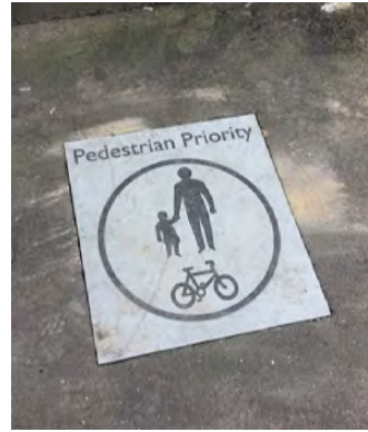
Fig 1.19 - Surface signage paver
