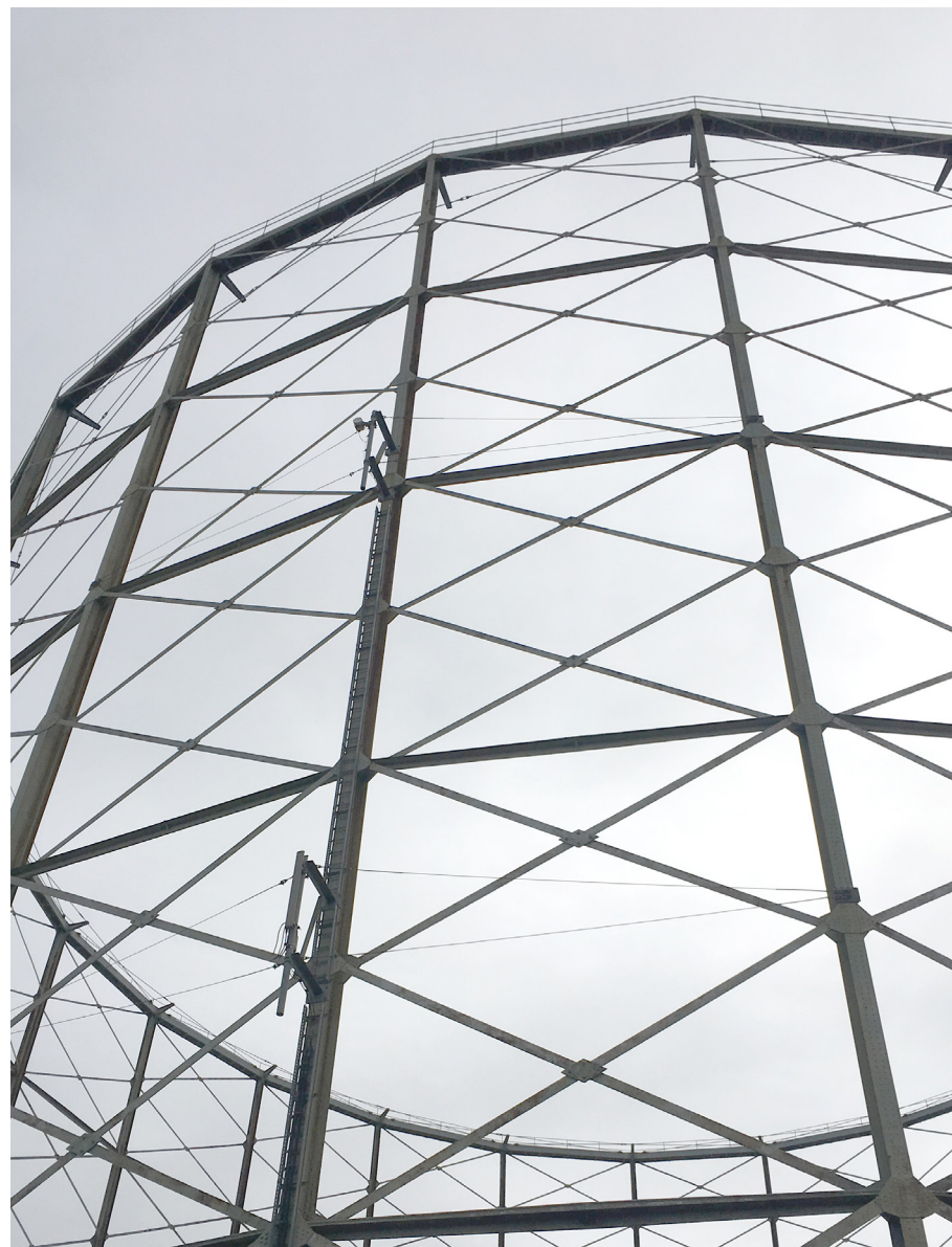
Figure 11: Detail of the structure of gasholder no.13
