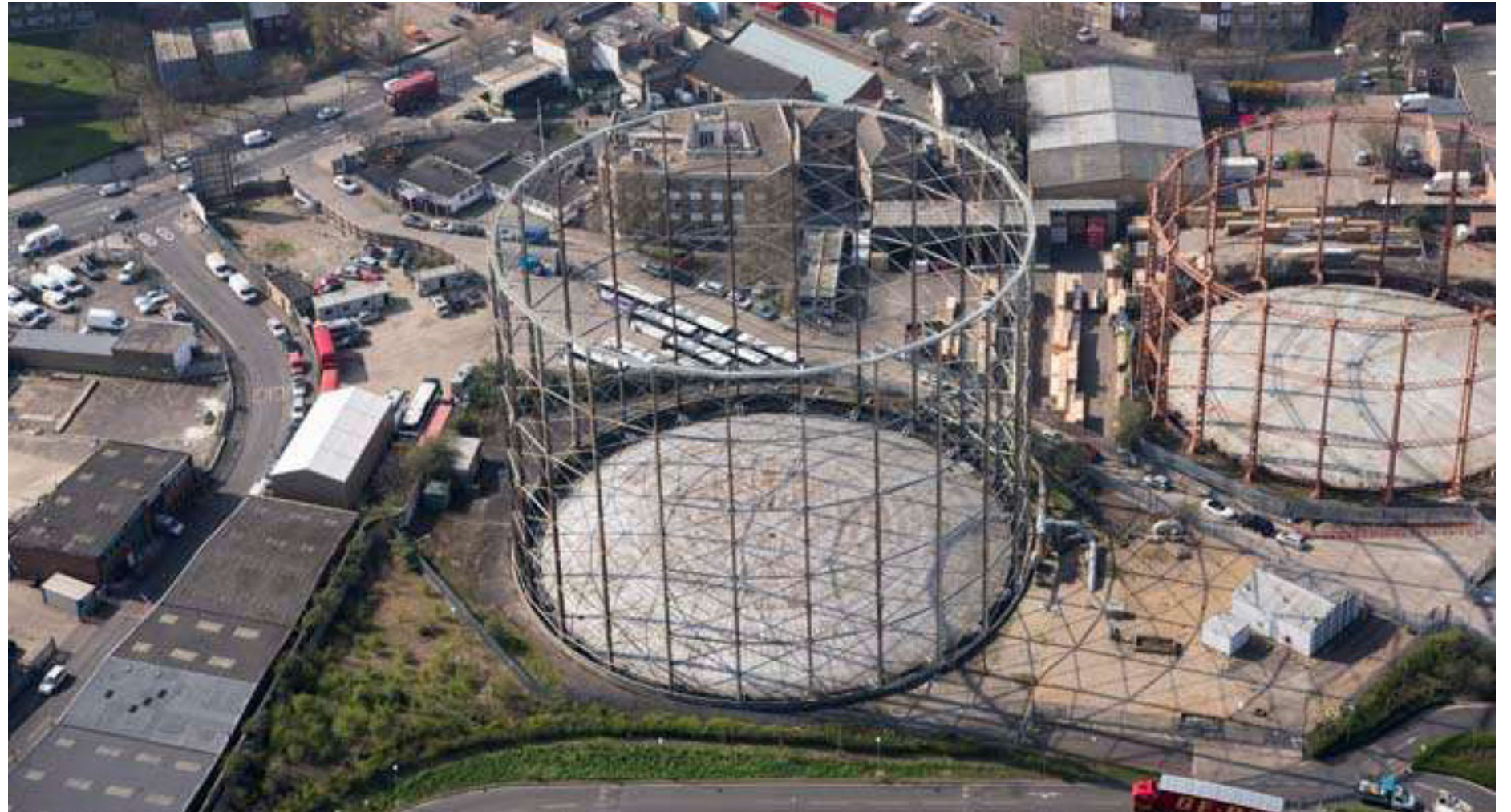
Figure 7: Aerial view of gasholder no.13
