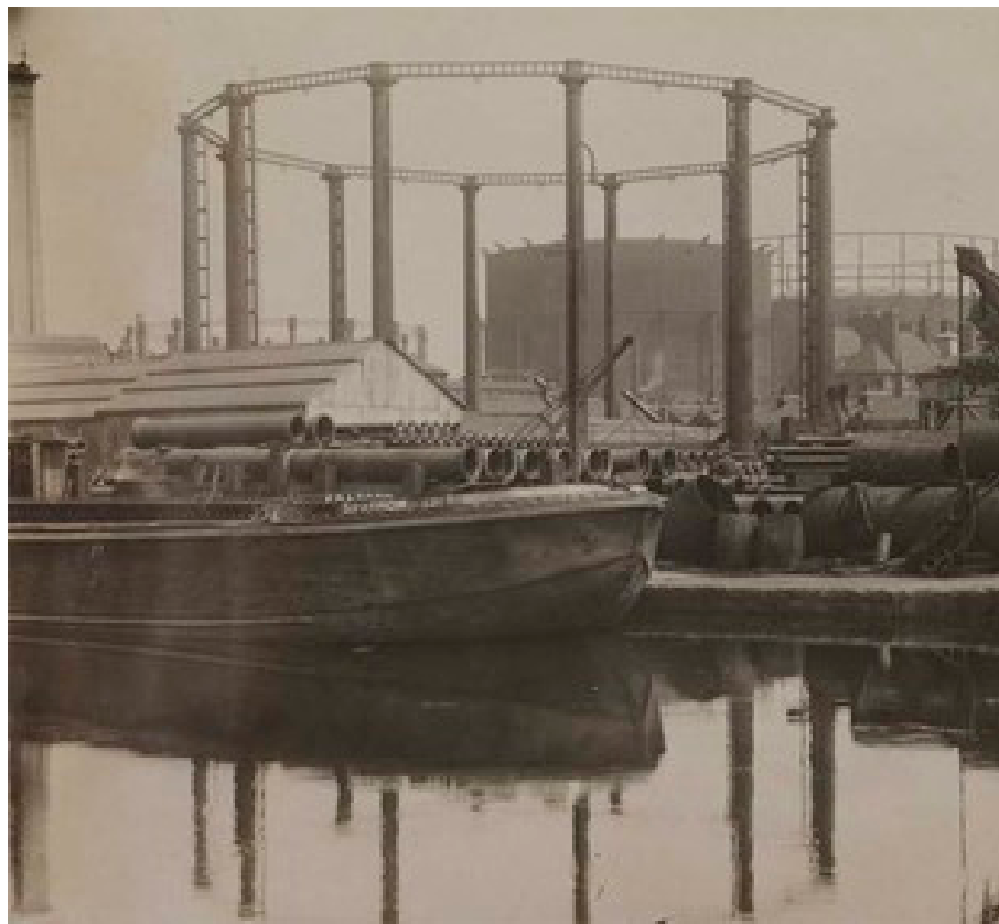
Figure 5: Historical image of the gasworks from the Surrey Canal
