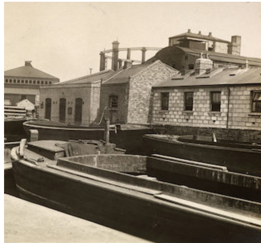
Figure 6: Historical image of the gasworks from the Surrey Canal
