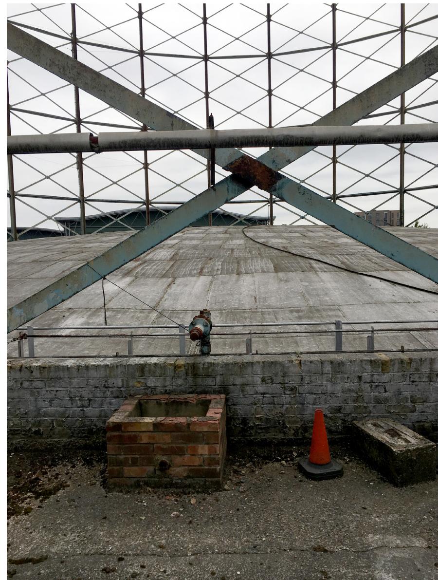
Figure 12: Detail of the tank dome of gasholder no.13
