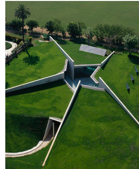
Figure 90: Gas pressure reduction station (3)
