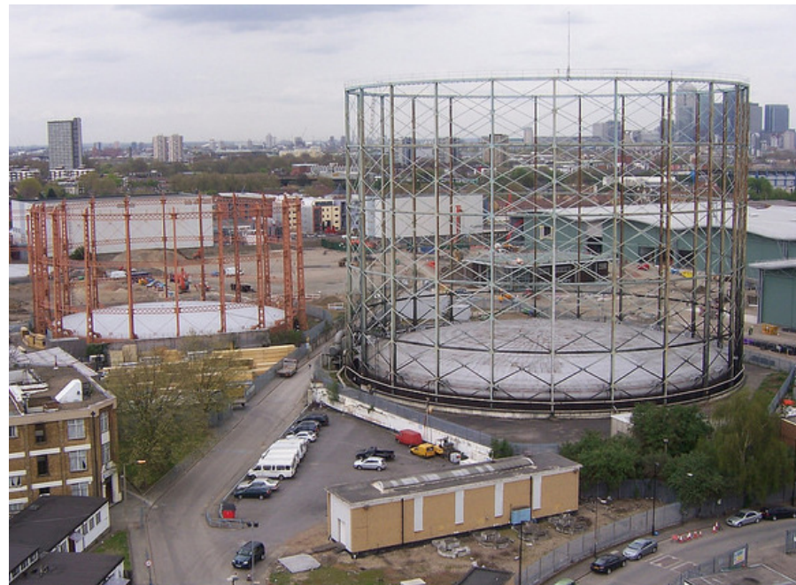
Figure 8: Aerial view of gasholder no.13
