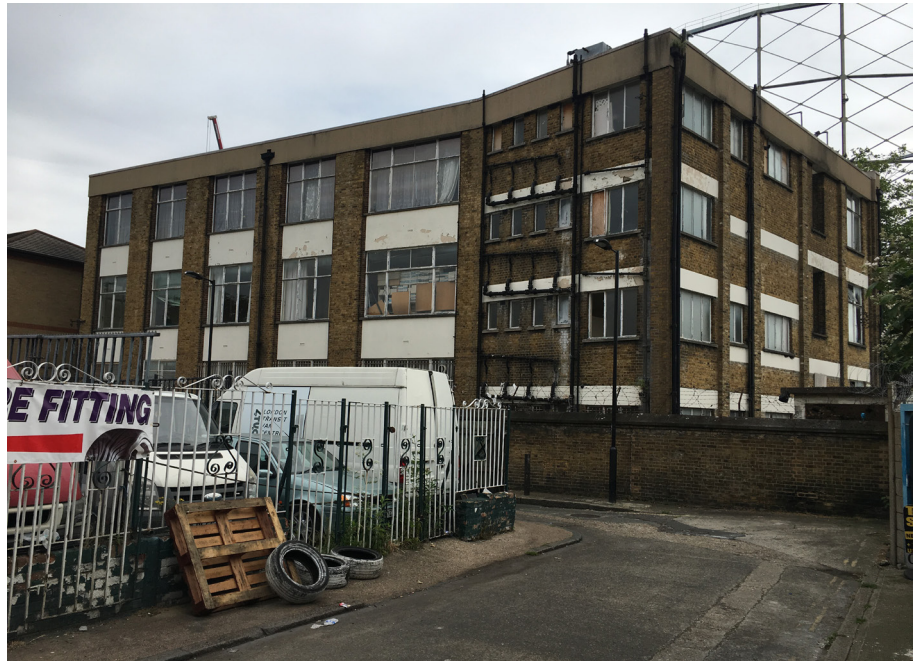
Figure 16: Office building to be retained
