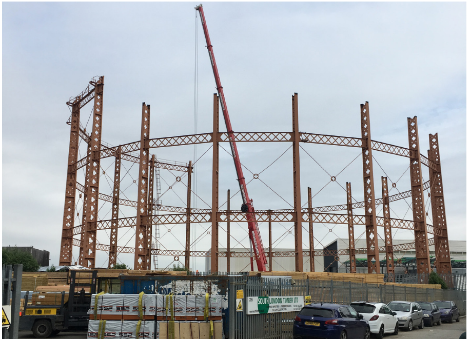
Figure 17: Gas holder no.12 being dismantled
