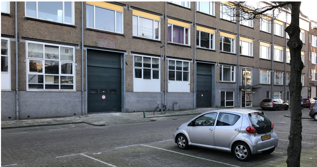
Small industrial units with residential above, Van Meekerenstraat, Rotterdam
