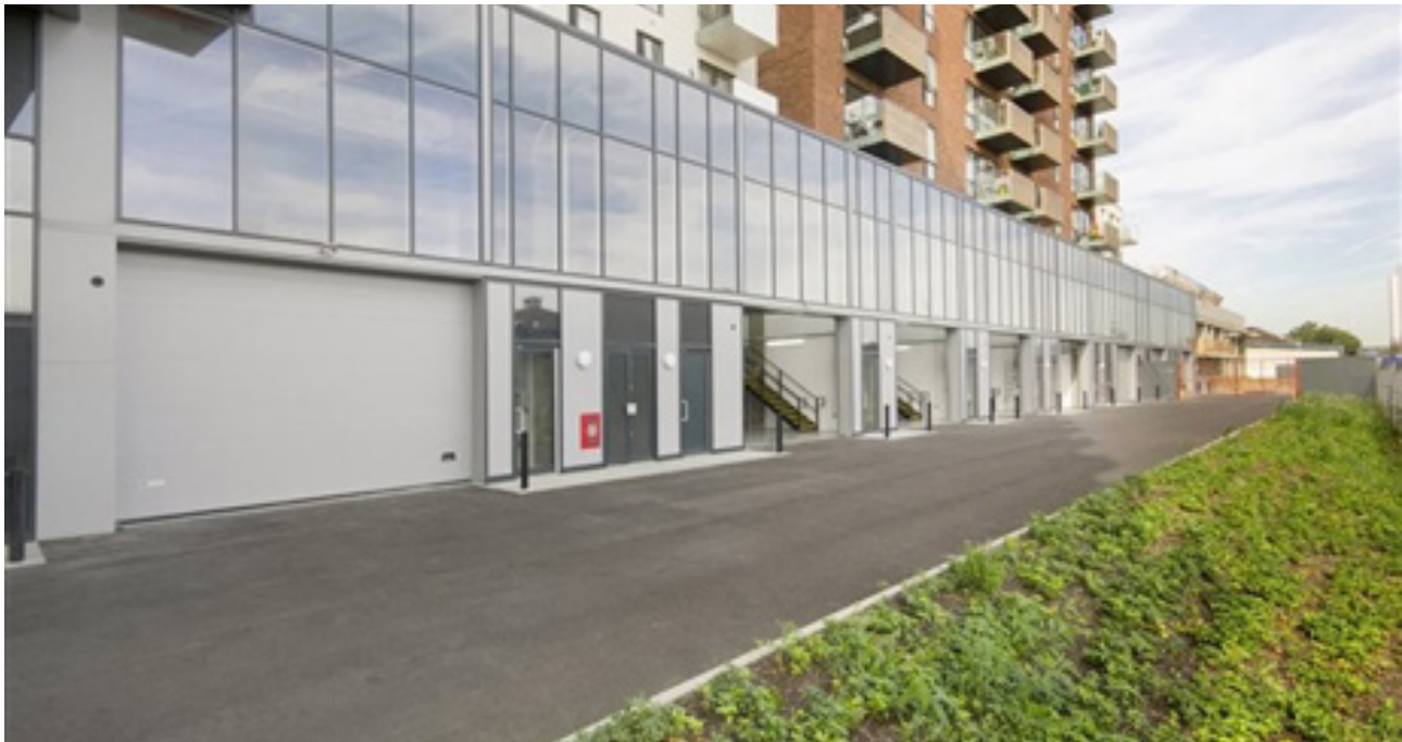
New light-industrial spaces with residential above, Bow Enterprise Park, London
