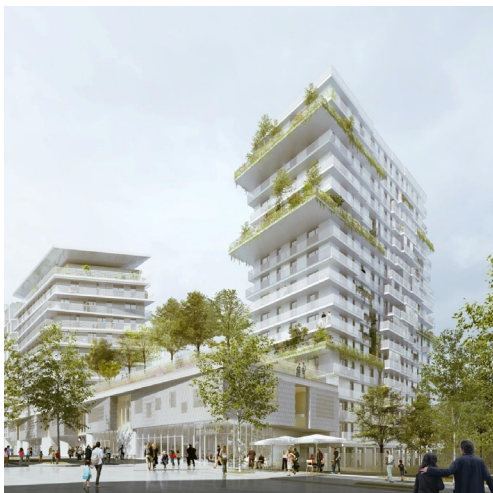
School integrated in residential block
