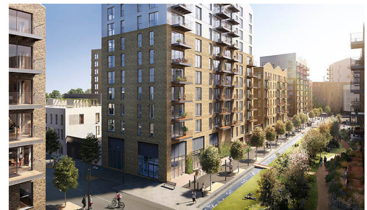
Deptford Wharf: A major new public space is created on the alignment of the former Surrey Canal at Deptford
