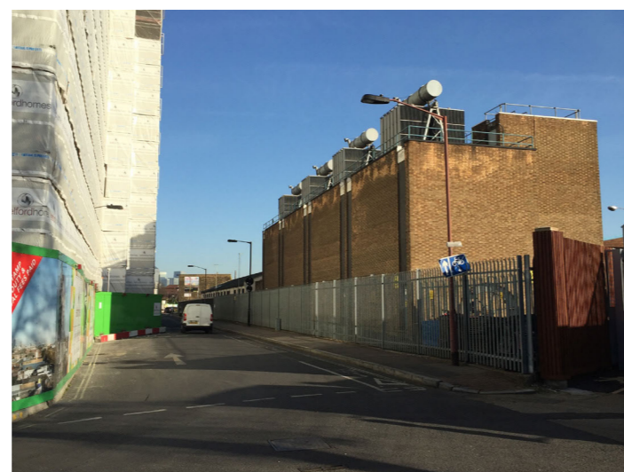
Existing sub-station to be retained along Verney Road
