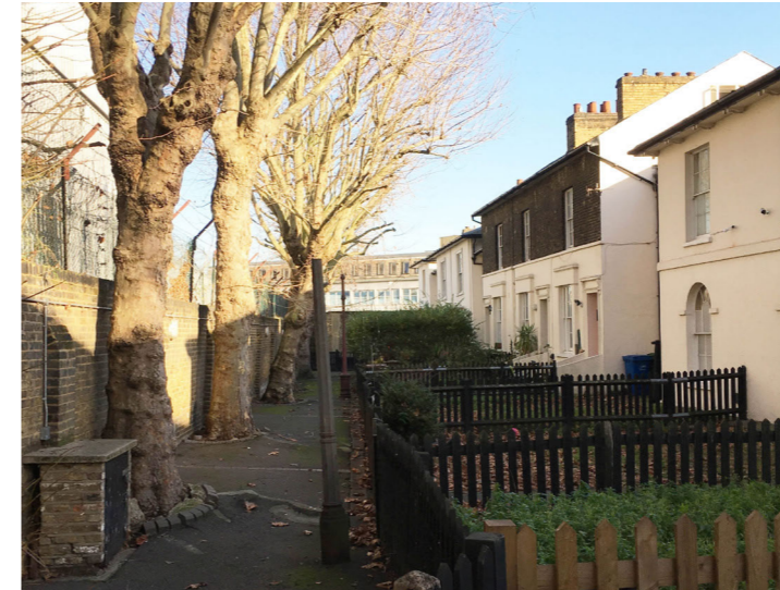
Listed houses tucked away within the site, linked to Old Kent Road via a poorly overlooked pedestrian link
