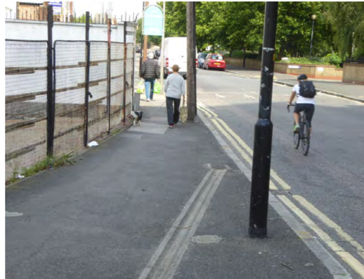
View 2 - The changing widths of the pavement are opportunities
