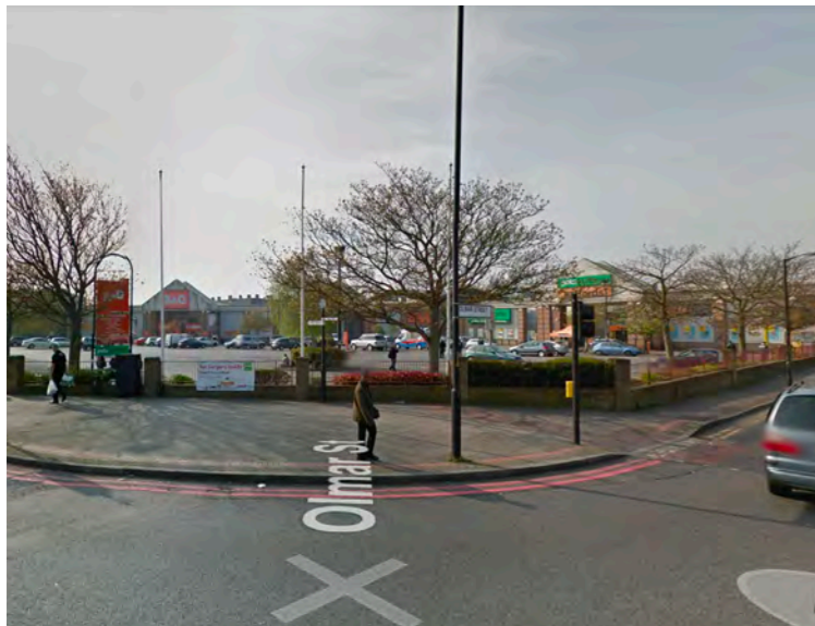
View 7 - Looking into the carpark to the left of Olmar street
