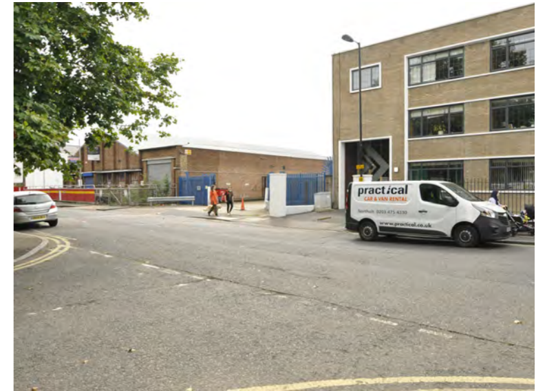
View 3 - The varied architectural character of St James's Road
