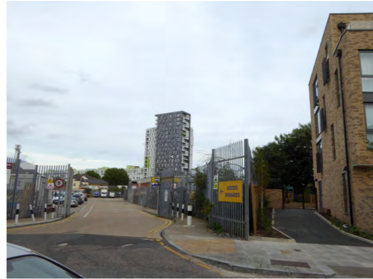
View 2 - The existing access point to the Six Bridges Industrial Estate
