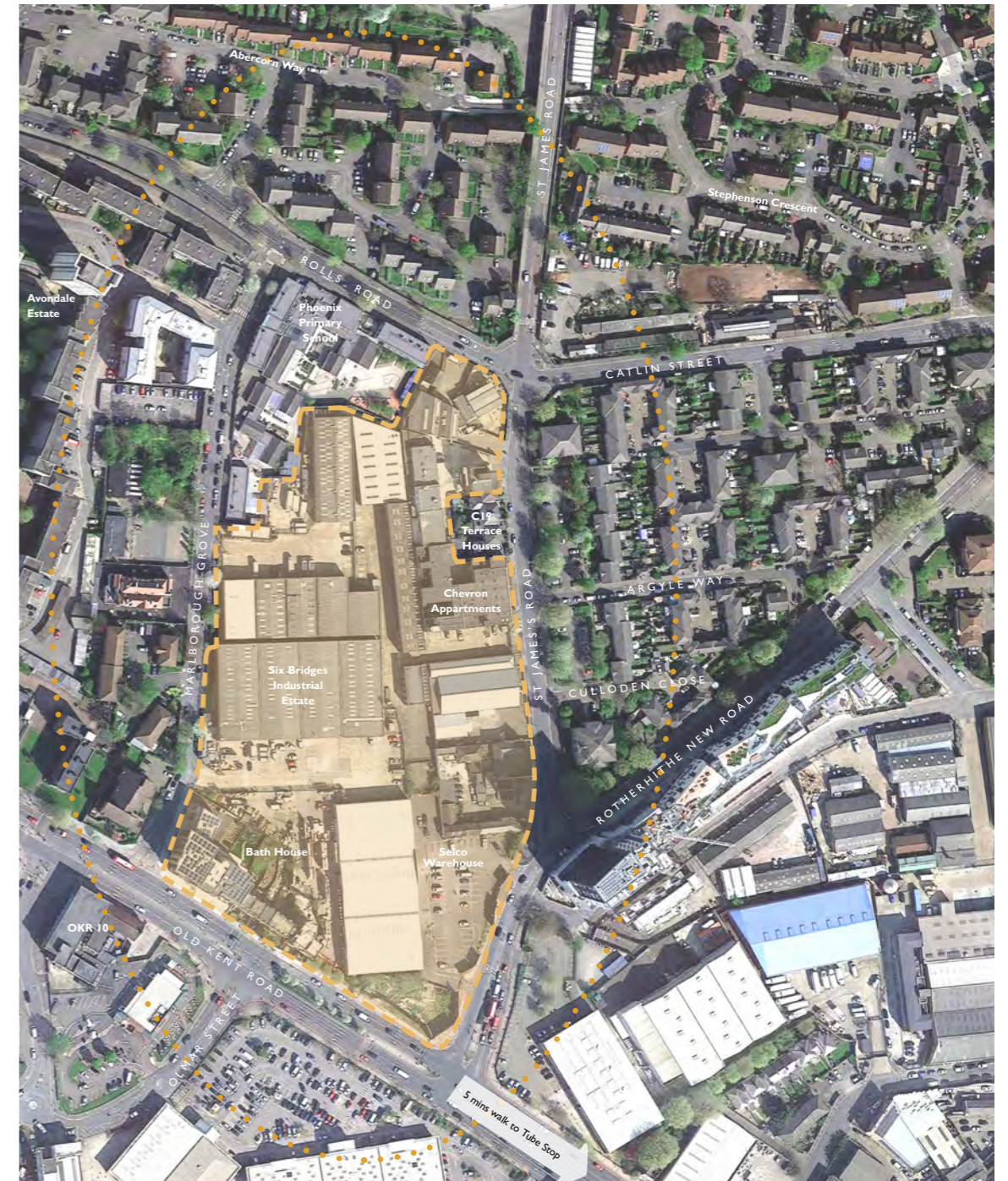
Aerial View showing the limit of OKR II
