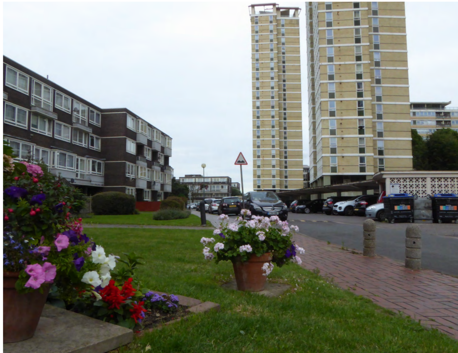
View 9 - Well cared for gardens of the Avondale Estate
