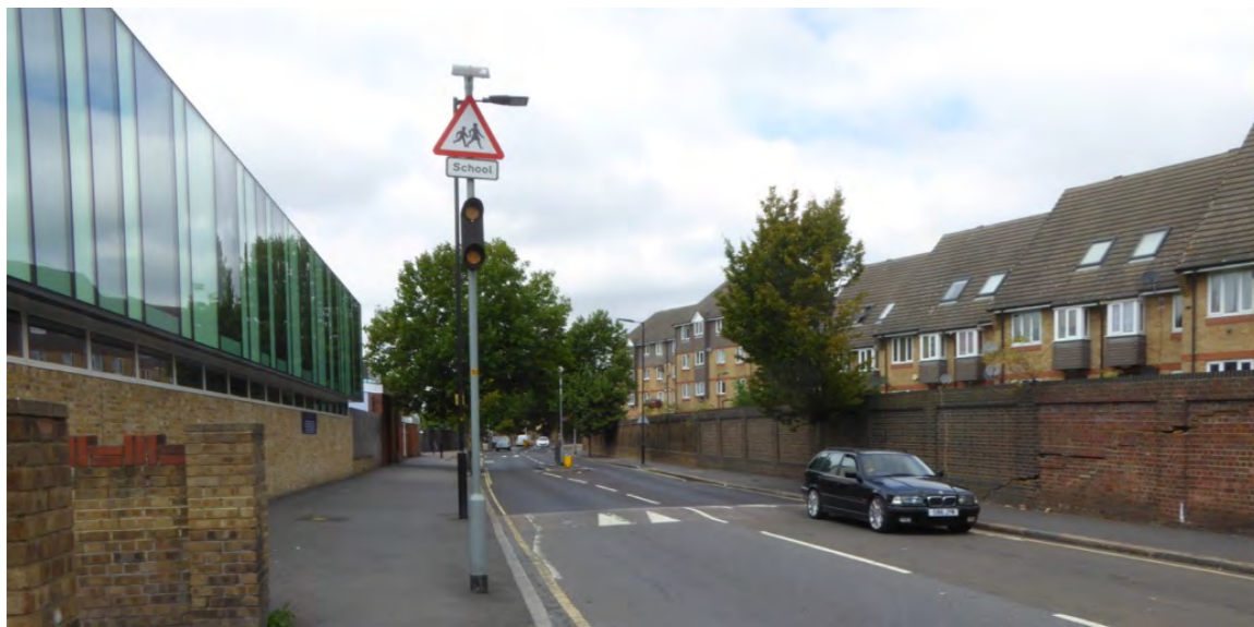
View 10 - Rolls Road is edged by an impermeable wall to the right, and an impermeable school building to the left
