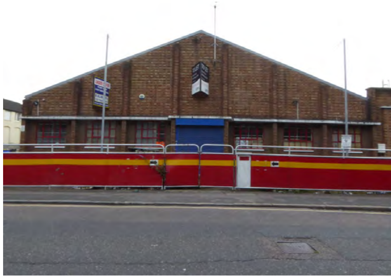
View 5 - Industrial buildings to be removed
