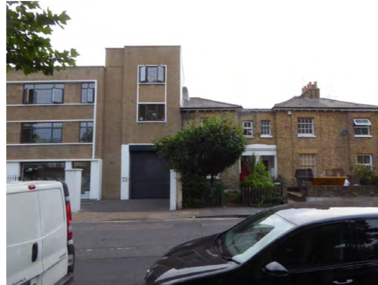
View 2 - The varied architectural character of St James's Road
