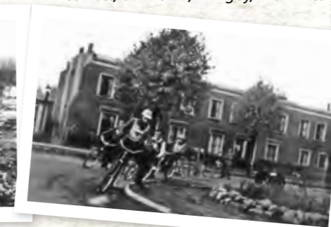
Lynton Lynx track looking to Lynton Road
