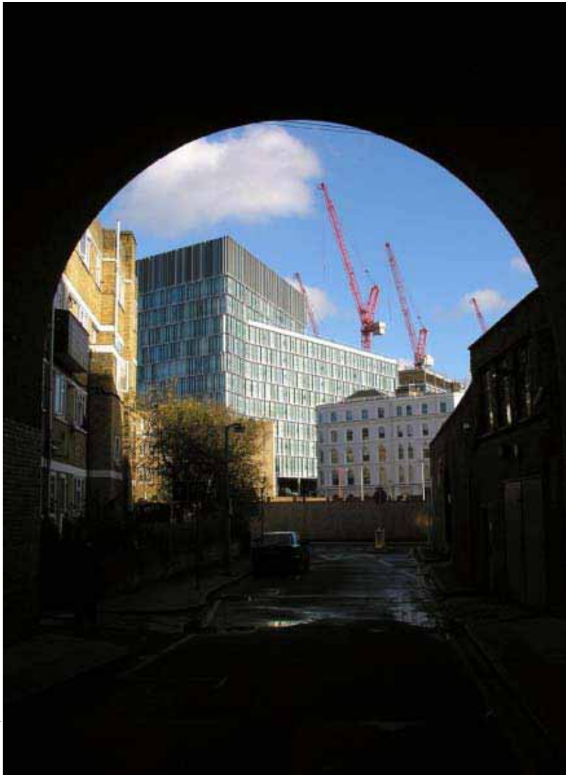
Blue Fin Building seen through Viaduct Arch
