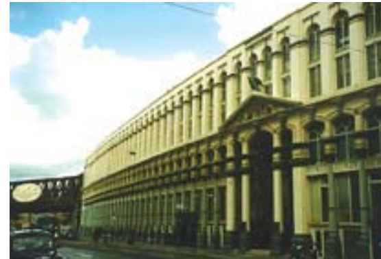
Figure 42 Hop Exchange, Southwark Street
