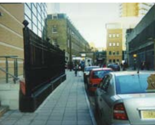
Figure 49 New Medical School frontage, Great Maze Pond, extending the strong building line of the east wing of the original Guy’s Hospital buildings.
