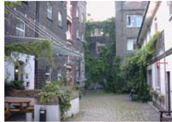
Figure 20 Original scale of yard retained in conversion of warehouses and workshops to new use: Axe and Bottle Court
