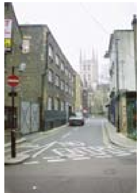
Figure 28 Winchester Walk is the main east-west link in the Cathedral area, with buildings such as no 16 defining a narrow street proportion and glimpsed views of the Cathedral.
