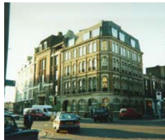
Figure 43 Portal of Borough Market and adjacent corner building, extending the curved building line of Southwark Street towards London Bridge.
