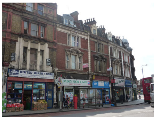
Nos.4-20 Camberwell Church Street: the distinctive elevations continue the detail of the listed Hartnell's building (No.2) with elaborate segmental arches, corbelled cornices and steep mansard attic roofs.
