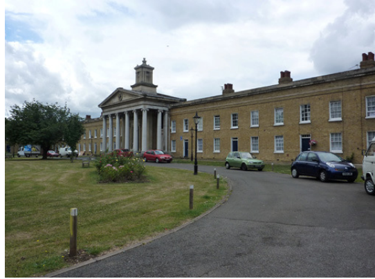
The Chapel at the centre of the composition, fronting the open space
