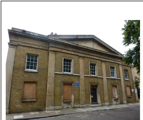
Boarded windows in the North Lodge
