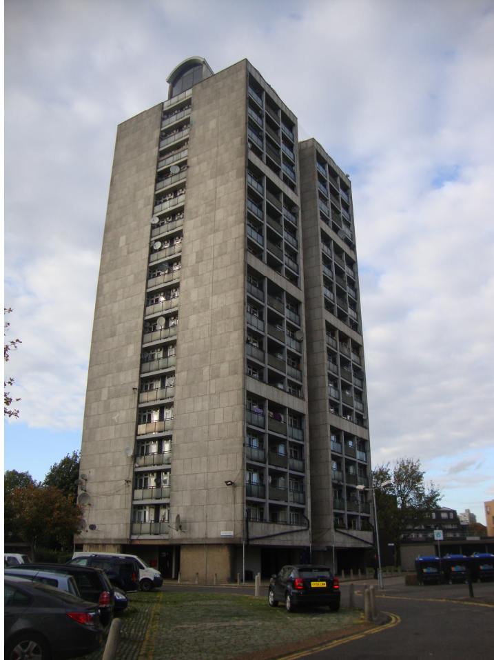
BATEMAN HOUSE (1-64) BRANDON ESTATE LONDON SE17
