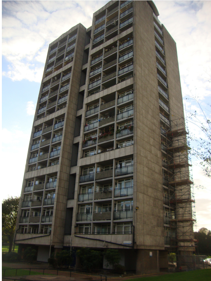
PRESCOTT HOUSE (65-68) BRANDON ESTATE LONDON SE17
