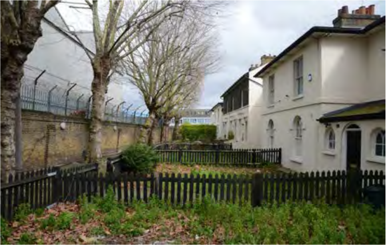
Grade II Listed Canal Grove Cottages, Old Kent Road
