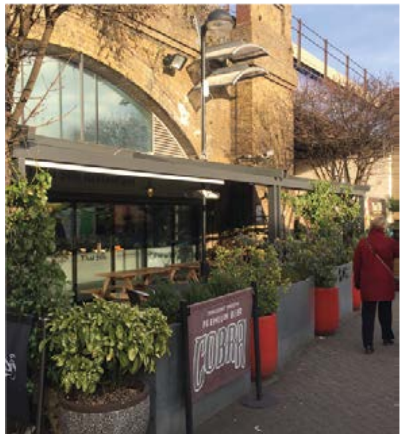
Railway Arches, Bermondsey Trading Estate
