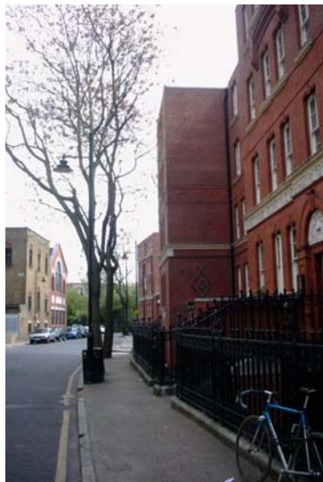
Figure 42 Guinness Trust Buildings, Snowsfields: showing the importance of the ensemble of railings, street furniture and trees in the character of the street.
