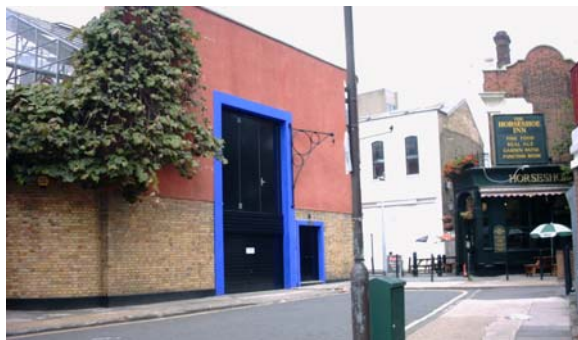
Figure 43 Melior Place: The Glasshouse Studio and The Horseshoe Inn contribute to a lively, local space.
