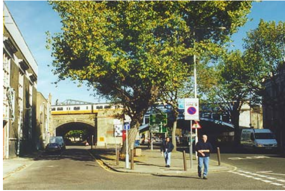
Figure 48 The Railway Bridge is a key element of spatial enclosure, related to the industrial architecture of the former Sarsons Vinegar works.
