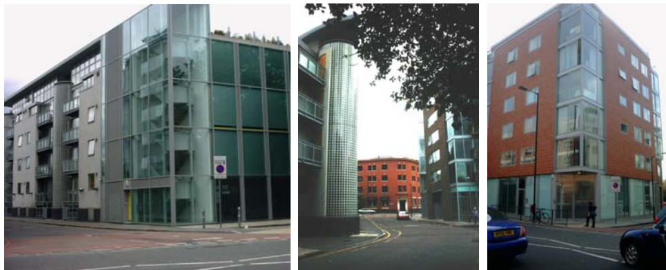
Figure 49,50, 51 New corner buildings on Tower Bridge Road.
