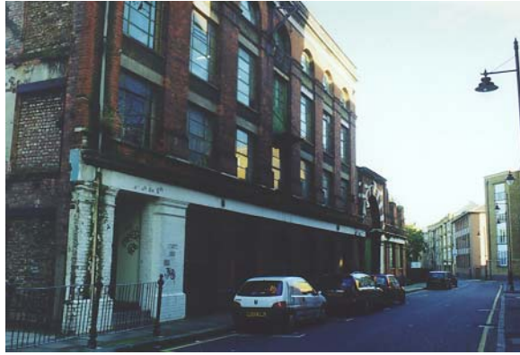
Figure 44 22, Leathermarket Street: former tannery in need of renovation, providing a counterbalance in the street scene to the impressive buildings of the Leathermarket Exchange, opposite.
