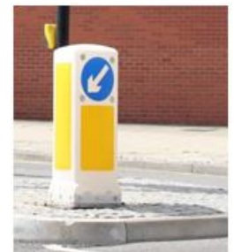
Illuminated bollard no longer used
