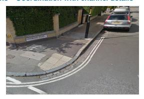
a. If a modular unit channel runs along the edge of a bituminous mixture surfaced carriageway then, where that detail is ≤ 300mm in width, waiting lines should be laid on the bituminous surface to the edge of the modular detail – not on the modular detail (see note). In other instances, (including where the entire carriageway is modular unit surfaced), the waiting lines should be laid on the channel detail. See standard DS.129 for further details.
