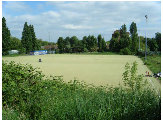
The artificial turf is coming to the end of its life span and is in a poor condition.
