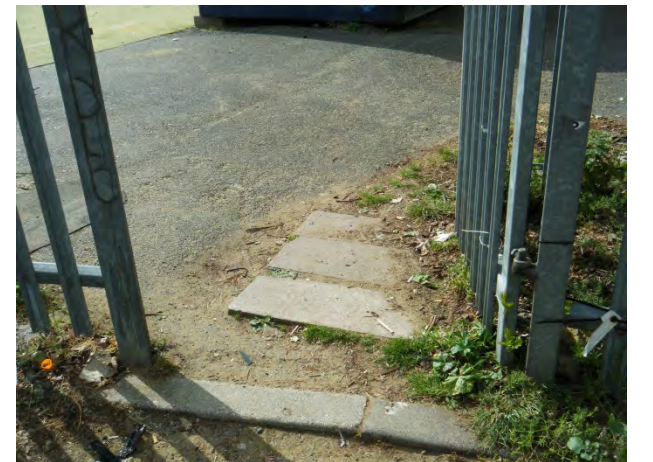
The pedestrian entrance to the artificial turf is uneven and narrow. The vehicle gates are padlocked. .
