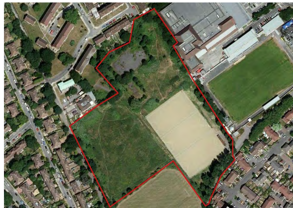
Figure 1.2 Aerial image of Greendale within the surrounding context
